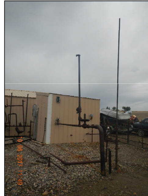
Photo 6. 2 – 1" steel risers not LO/TO.
