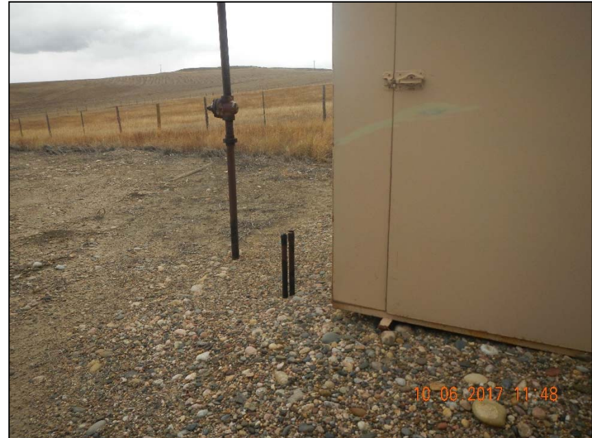
Photo 4. 2 – 1" steel risers not LO/TO.
