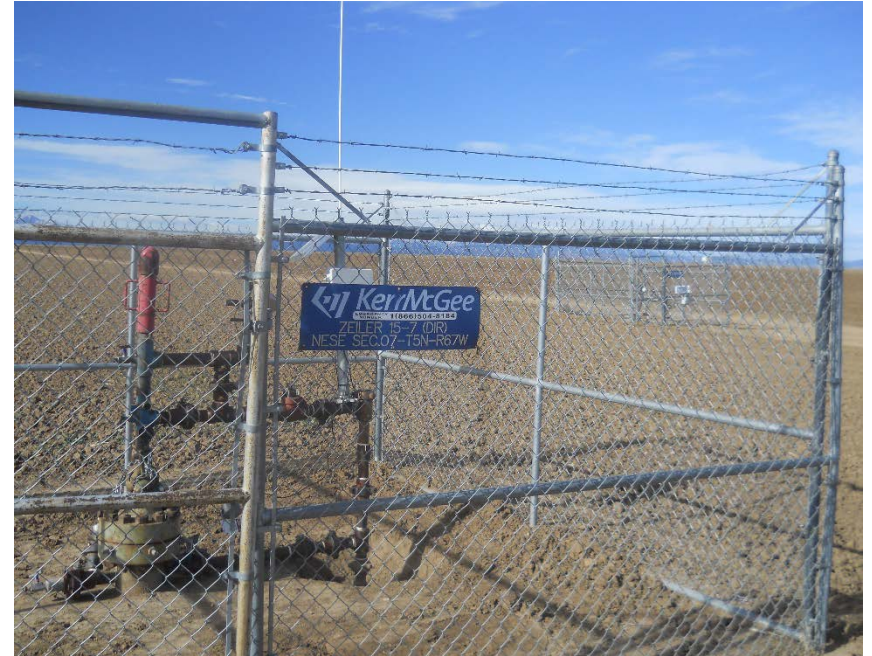
Unused methanol tank and fencing has been removed from Zeiler 15-7 wellhead
