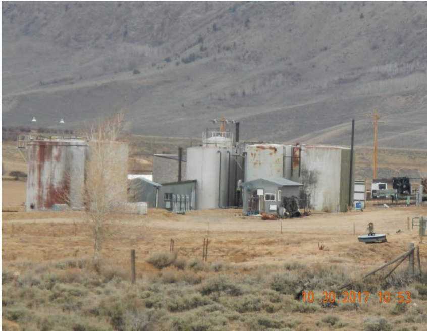
Centralized Tank Battery
