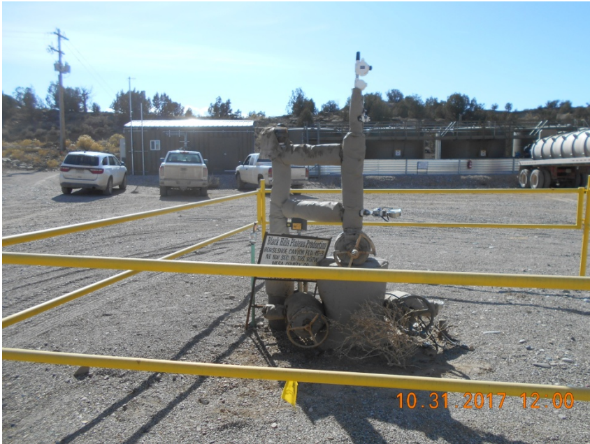
Wellhead and facilities. 1" service riser at wellhead (point A).
