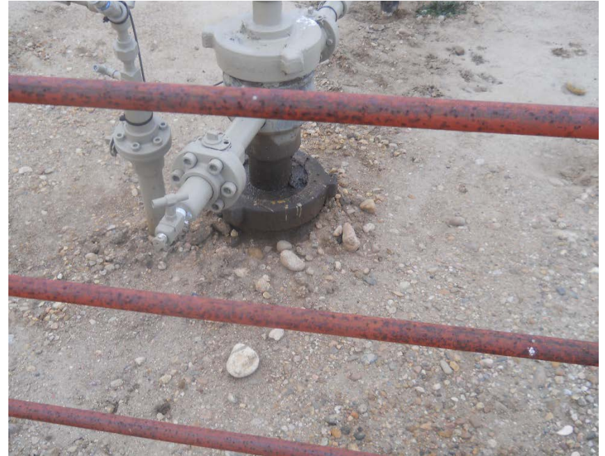
Stained soil around wellhead needs to be cleaned up
