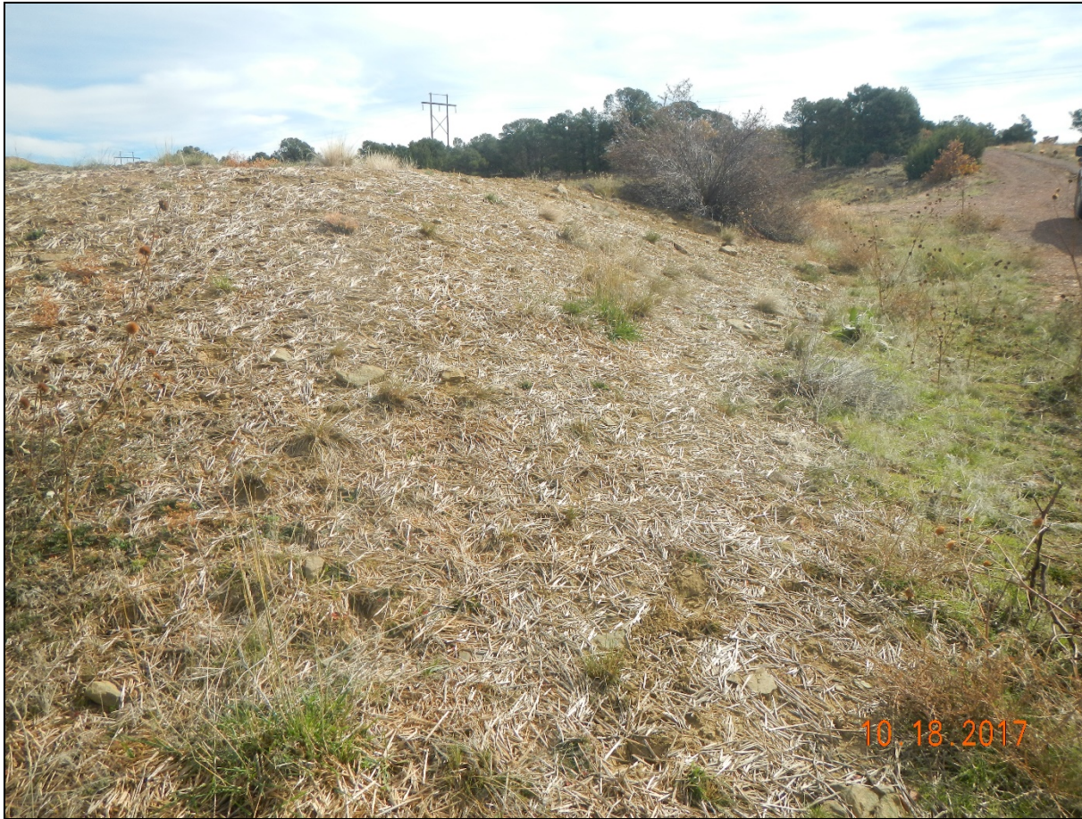
Photo 9. Facing southeast along the fill slope. Wood mulch has been applied along the fill slope.
