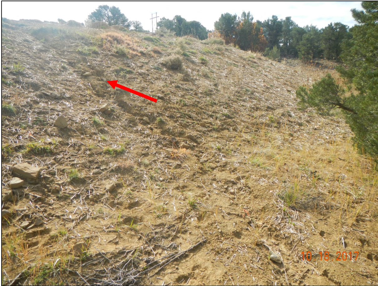
Photo 8. Facing toward the fill slope. There is signs of erosion occurring off the fill slope.
