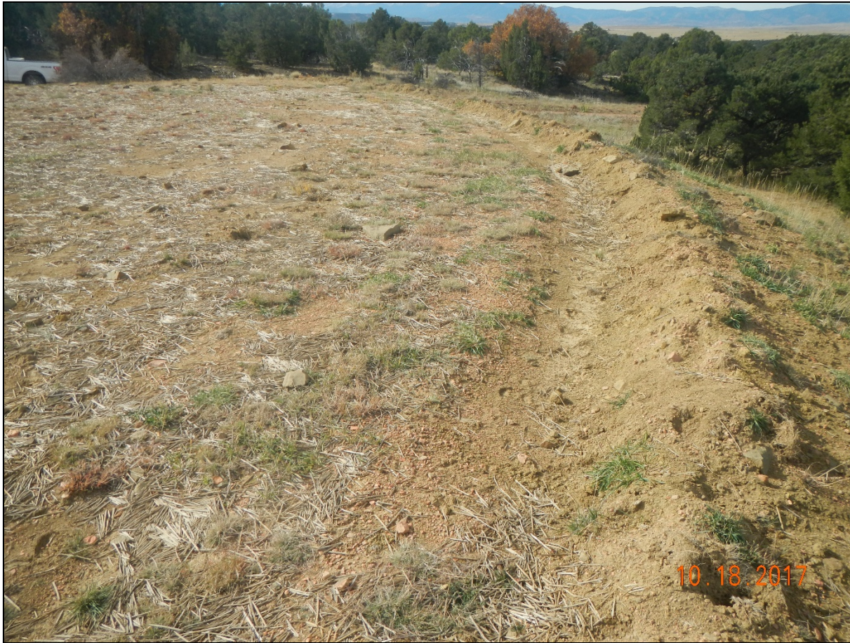
Photo 6. Facing west along the cut slope. A berm has been placed at the edge of the pad.
