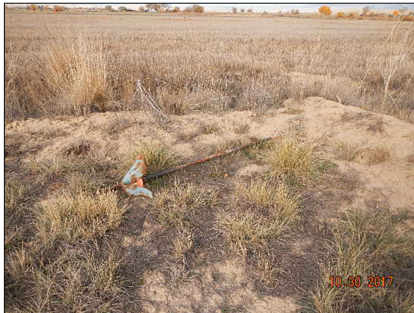
Photo 2. One of two unused deadman anchors.
