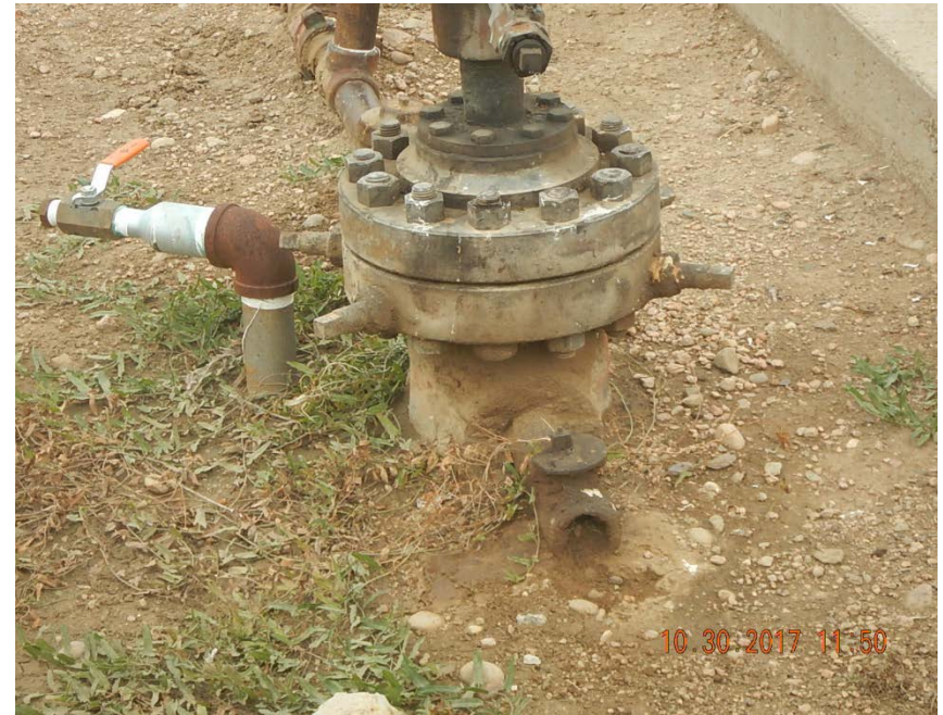
Photo 3: Bradenhead plumbed to surface, stained soil removed
