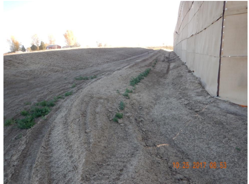
Photo 4. Photo taken from the northwest location, facing East. See comments under Photo 3. Topsoil salvaged and stored along the northern perimeter.
