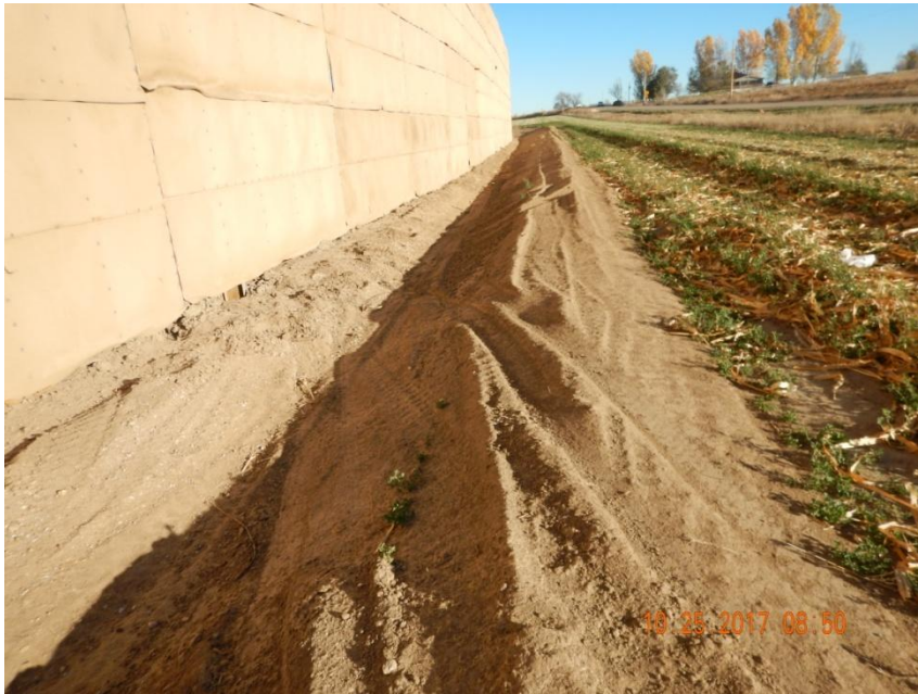
Photo 3. Photo taken from the southeast location, facing North. Ditch and berm BMP installed around the perimeter of the location. Appears hydromulch has been applied to the ditch and berm BMP to temporarily stabilize BMP.
