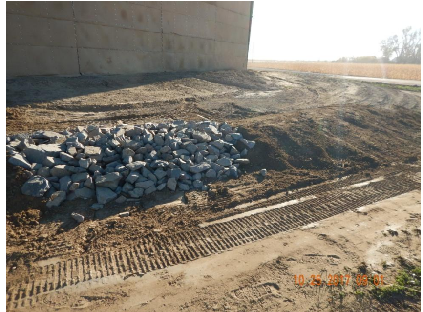
Photo 6. Photo taken from the southwest location, facing Southeast. Retention area constructed along the southwestern location with a stabilized outlet device.
