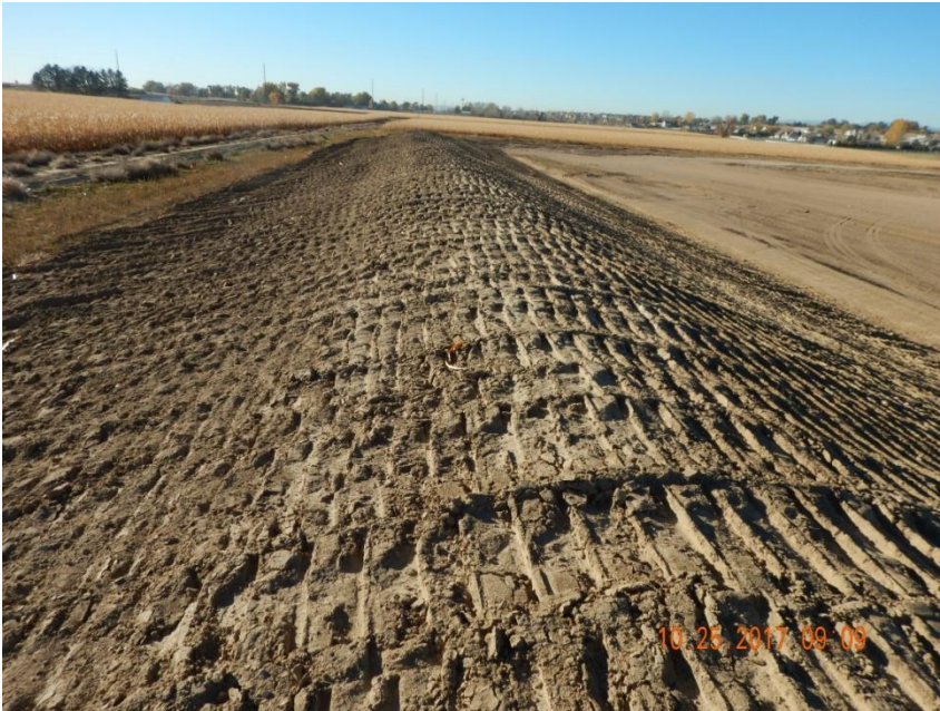
Photo 1. Overview photo taken from the eastern location, facing South. Topsoil salvaged and stored along the eastern perimeter of the location.
