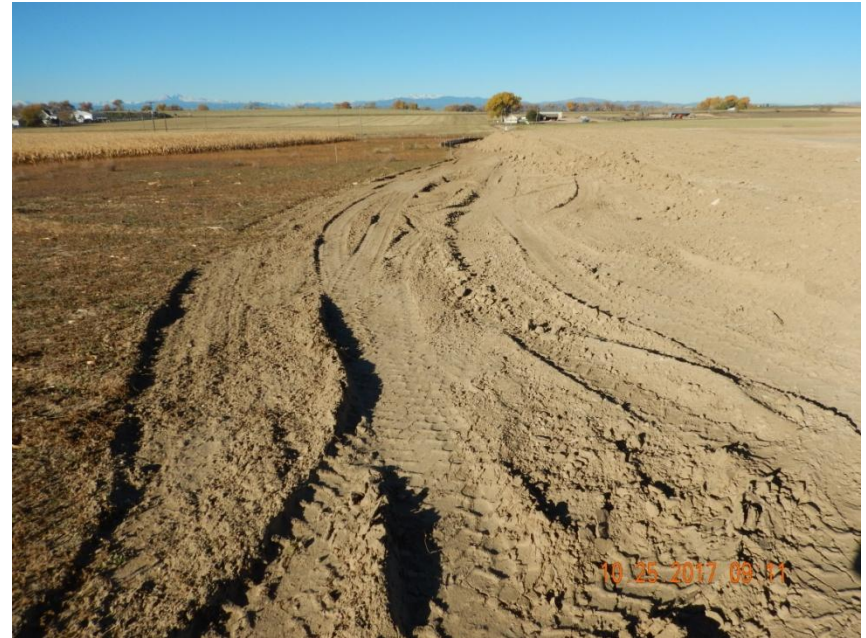
Photo 6. Photo taken from the southeastern location, facing West. No stormwater and erosion control BMPs observed along this portion of the location. Operator plans to install ditch that will be directed to the sediment basin which has already been constructed.
