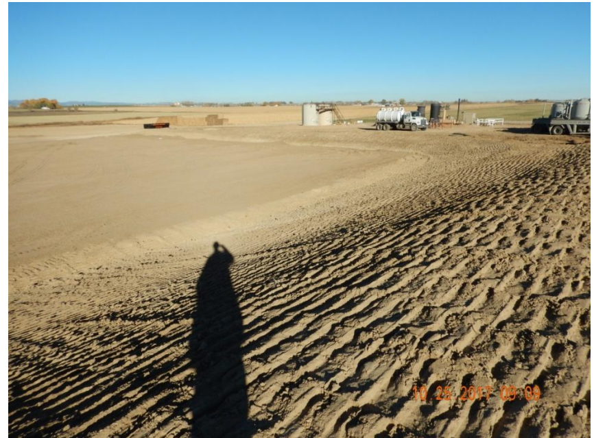
Photo 4. Overview photo taken from the eastern location, facing Northwest. See comments under Photo 1.
