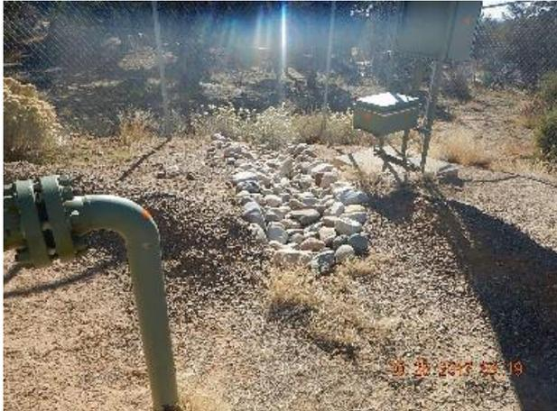
Photo 7: Installed rip rap and sediment trap in SE corner.
