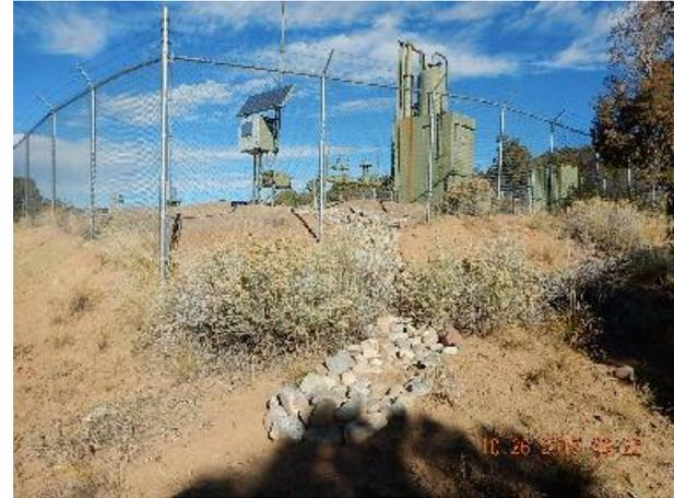
Photo 8: Installed rip rap and sediment trap in SE corner from outside the fencing.
