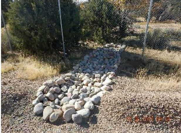
**Photo 5: Installed rip rap and sediment trap on S edge of location.**
