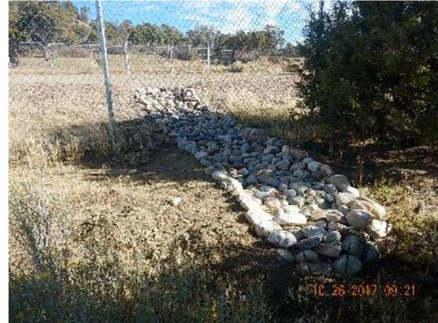
**Photo 6: Installed rip rap and sediment trap on S edge of location view from outside fencing.**
