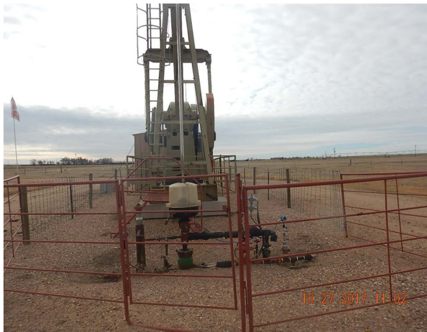
Photo 1: Wellhead, looking S
