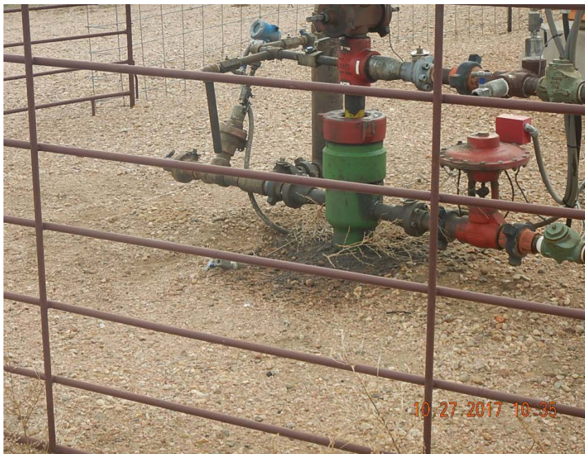
Photo 3: Stained soil at wellhead
