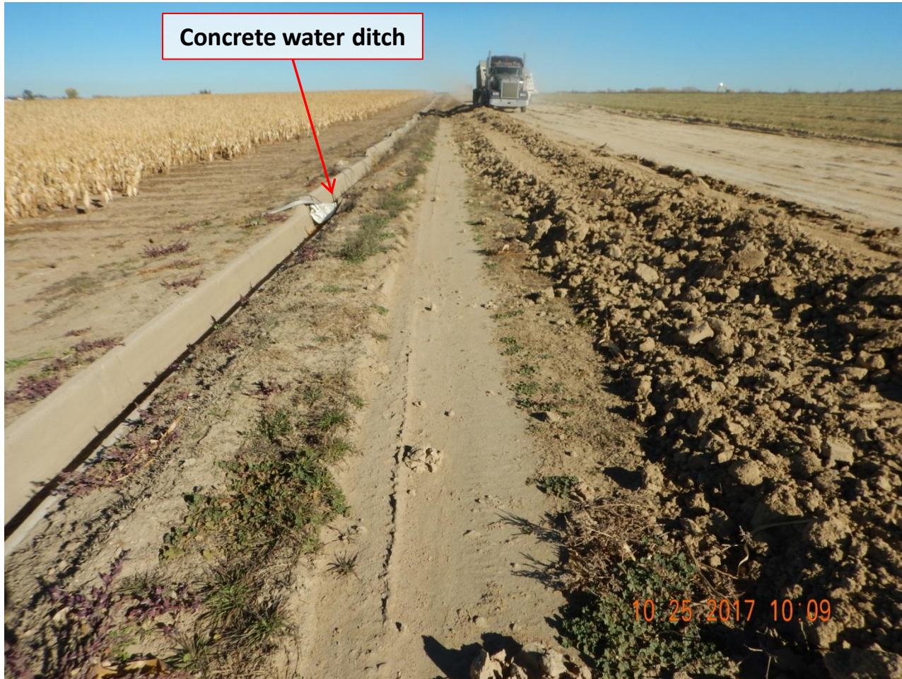
Photo 7. Photo taken from the access road, facing North. Operator shall stabilize unconsolidated soil material along the access road.
