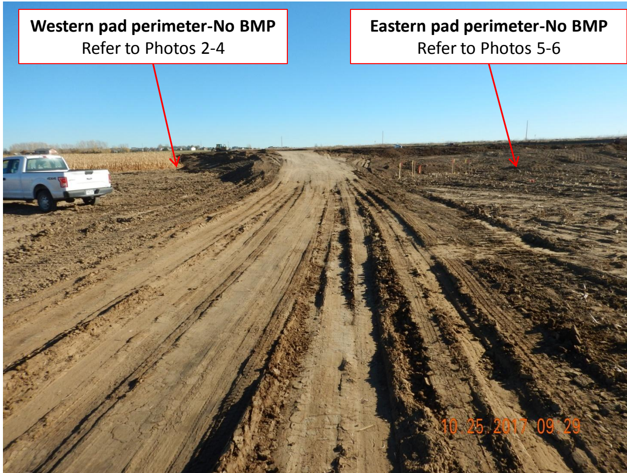
Photo 1. Photo taken from the entrance of the location, facing Northeast. No stormwater or erosion control BMPs were observed throughout any portion of the location. Per Form 42 (Notice of construction), construction activities commenced on September 18, 2017. Operator has failed to install stormwater and erosion control BMPs prior to, or at, the start of construction.
