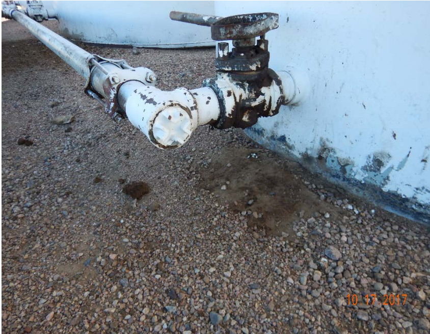
Photo #19 – Localized historical accumulation of oily waste and oil-stained soil beneath 300 bbl crude oil AST loadout valves (1).
