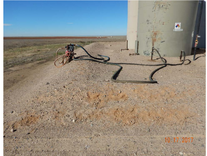
Photo #28 – Shallow/damaged earthen berms at SE corner of crude oil tank battery.
