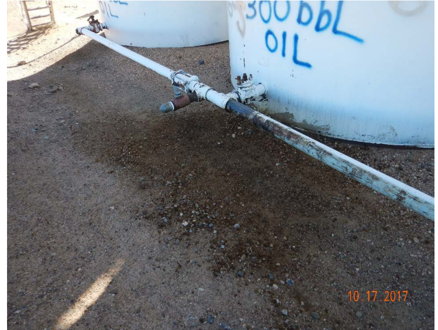
Photo #20 - Localized historical accumulation of oily waste and oil-stained soil beneath 300 bbl crude oil AST loadout valves (2).
