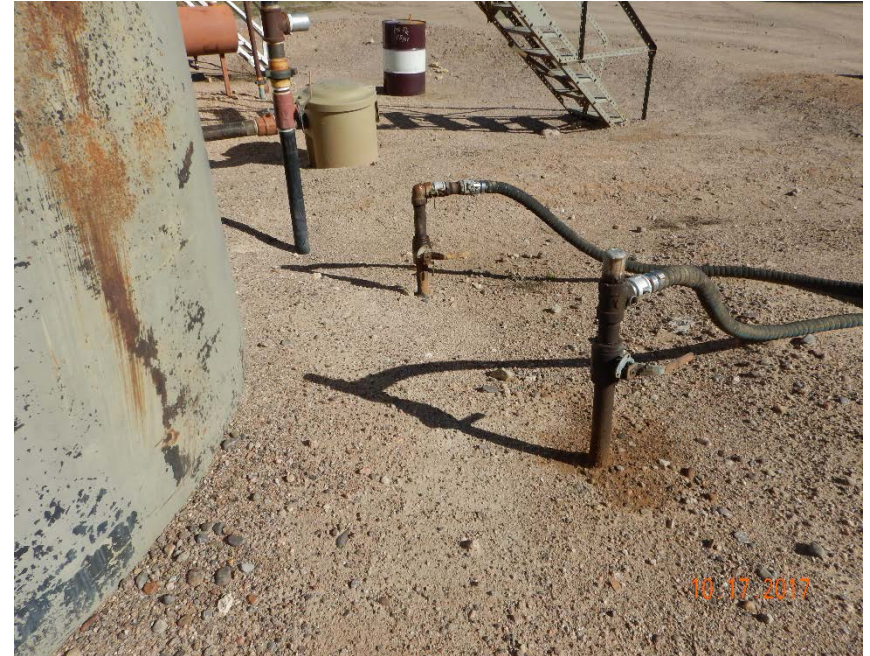
Photo #26 – Active 2" flowline risers with localized, oil-stained soil located east of 400 bbl crude oil ASTs.
