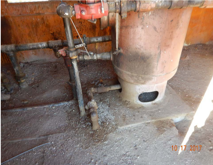
Photo #15 - Localized, historical accumulations of oily waste inside of Wickstrom #6-5 treater/separator shed (2).
