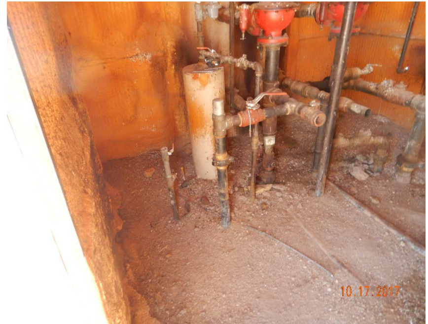
Photo #14 – Localized, historical accumulations of oily waste inside of Wickstrom #6-5 treater/separator shed (1).
