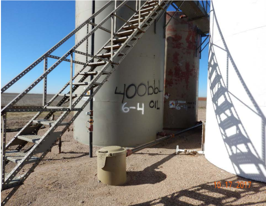
Photo #23 – 400 bbl crude oil ASTs south of 300 bbl crude oil ASTs.
