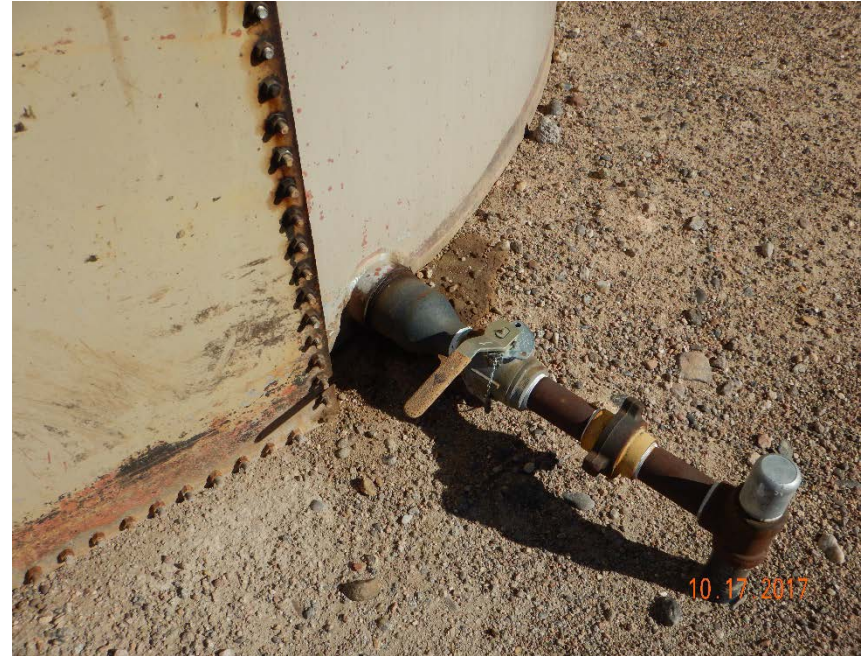
Photo #24 – Localized, oil-stained soil beneath valve on south side of 400 bbl crude oil AST.
