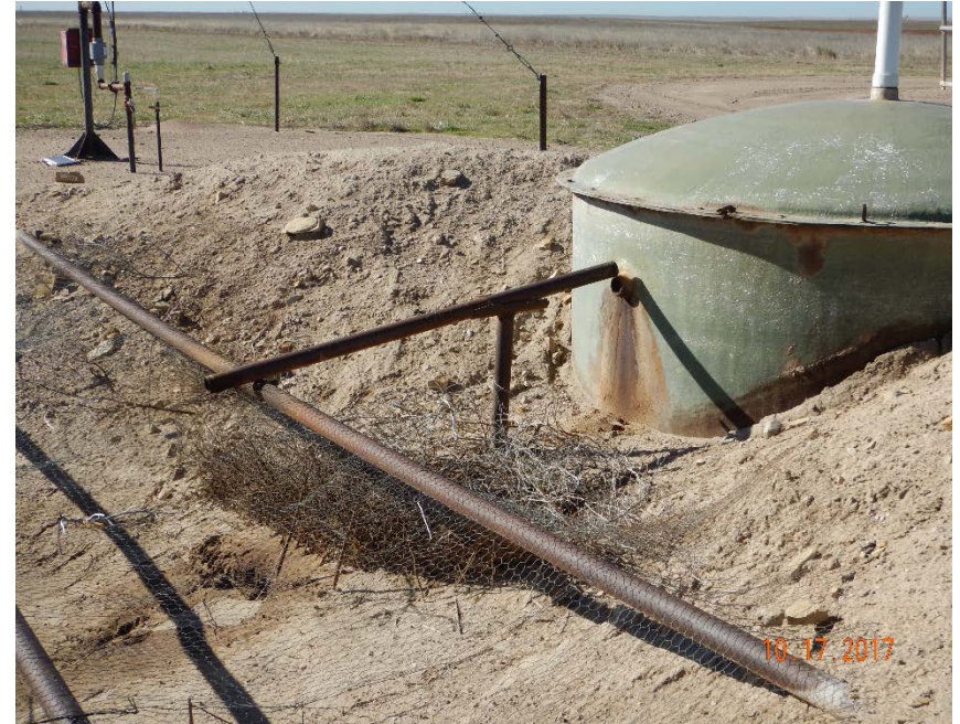
Photo #30 – Skim tank outlet to pit is disassembled. Note: oil-stained soil and weeds at skim tank outlet.
