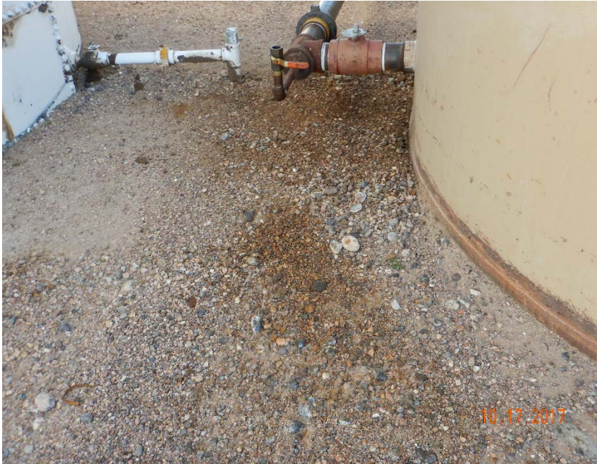
Photo #25 – Localized, oil-stained soil beneath valve on north side of 400 bbl crude oil ASTs.
