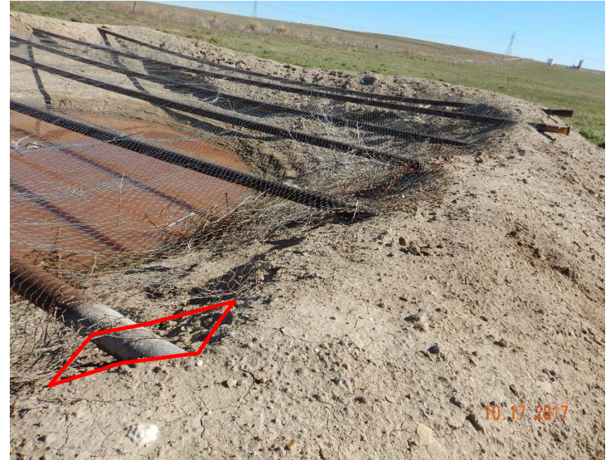
Photo #34 - Gaps in mesh cover for produced water pit (2).
