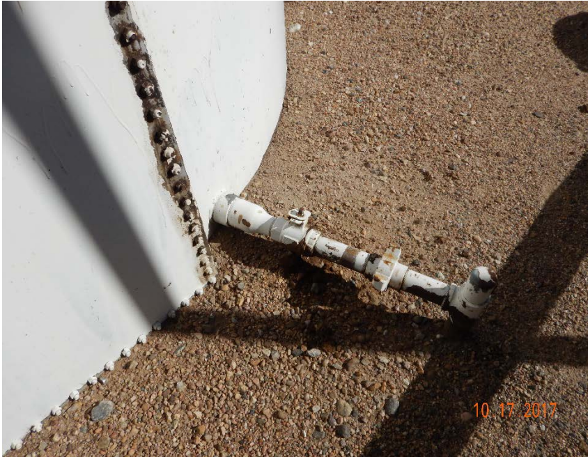
Photo #21 – Localized, oil-stained soil beneath valve on south side of 300 bbl crude oil AST.
