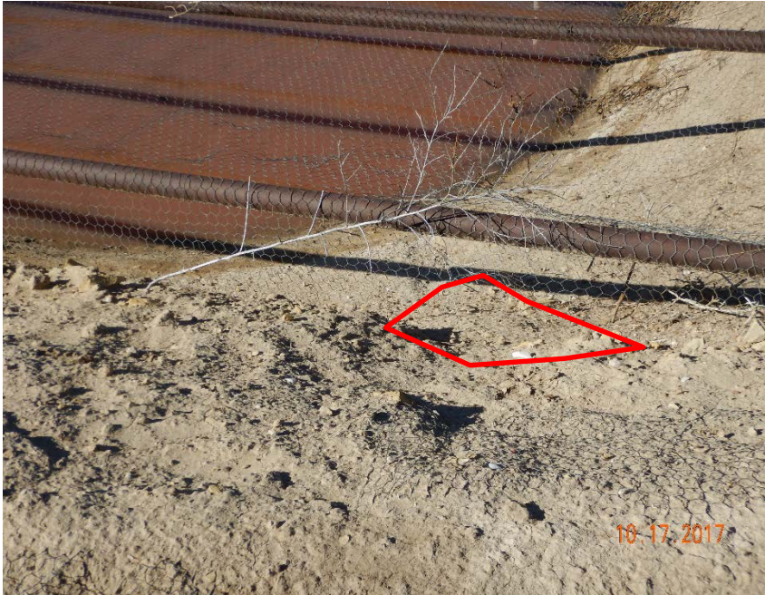
Photo #33 – Gaps in mesh cover for produced water pit (1).
