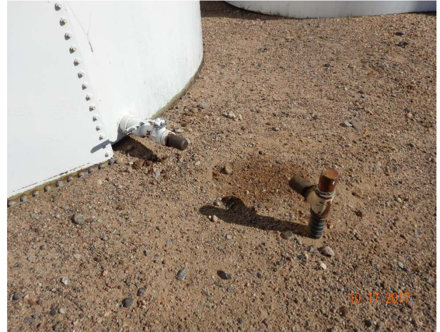
Photo #18 – Unused flowline riser with localized, oil-stained soil on south side of western 300 bbl crude oil AST.
