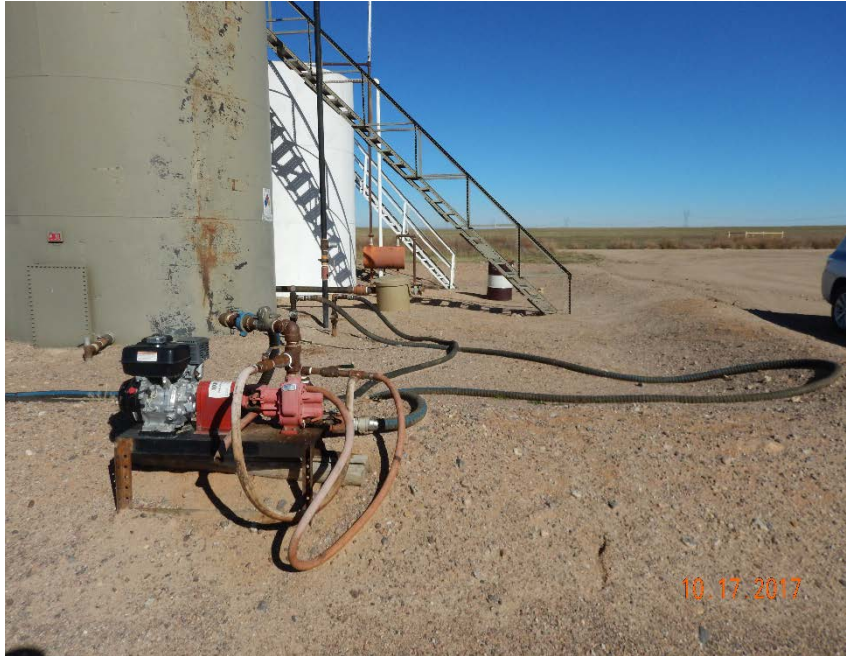
Photo #27 – Gas-powered pump plumbed to active flowline risers at SE corner of crude oil tank battery.
