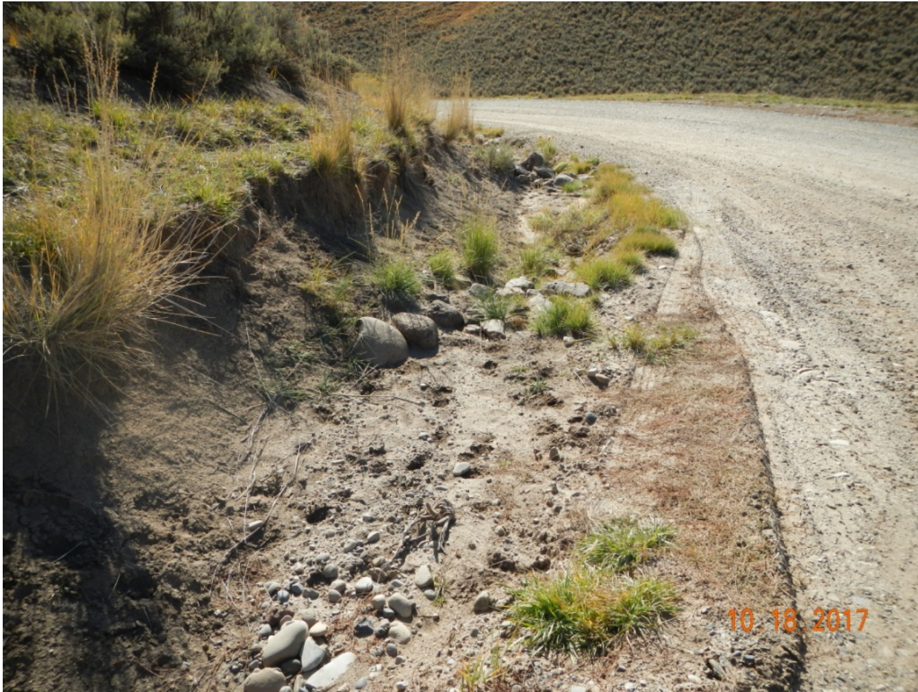
Photo 5. View of rock check dams along the access road that are full of sediment and need maintenance.
