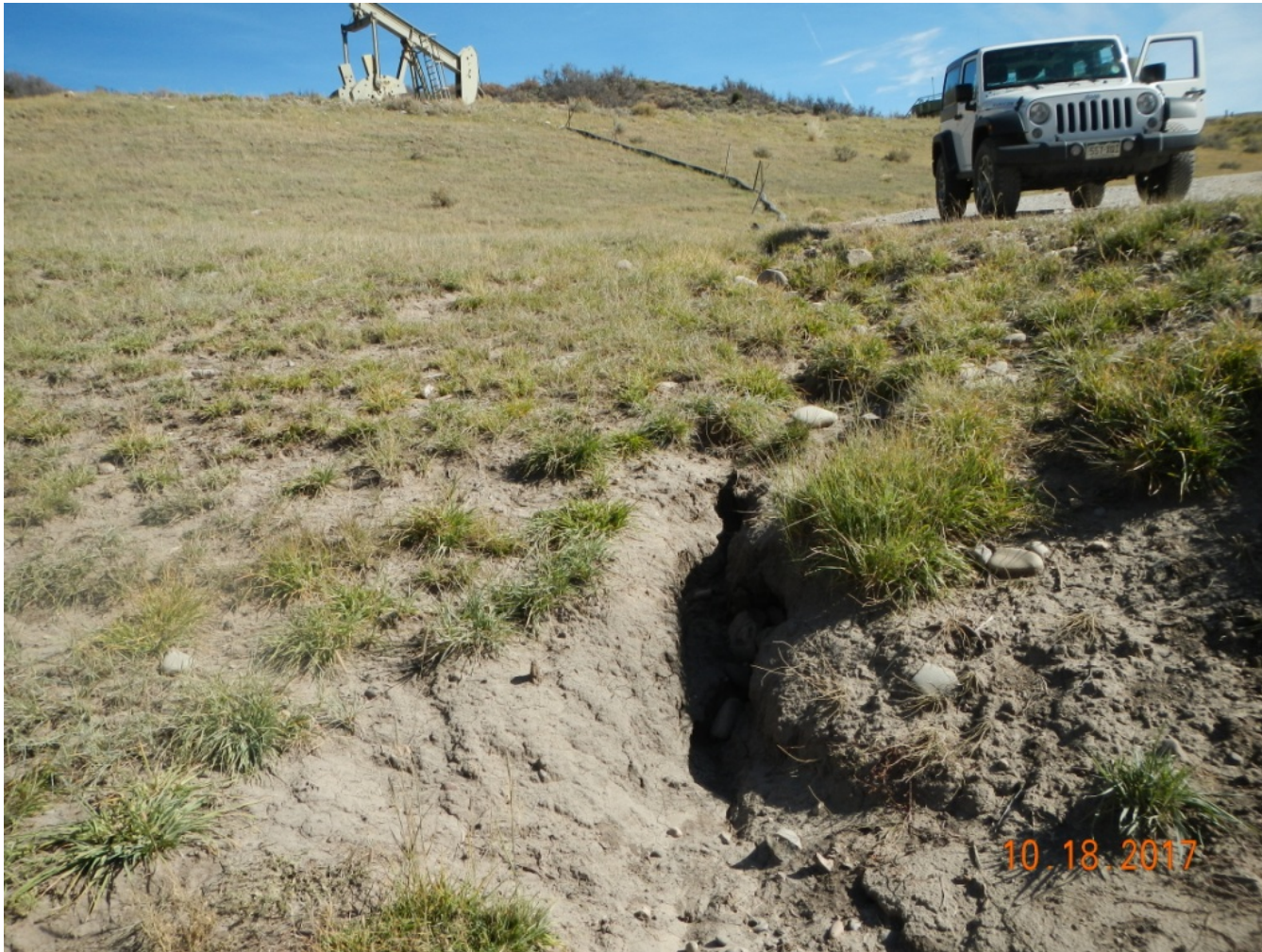
Photo 6. View of erosion that is occurring where concentrated stormwater exits a black pipe diversion from the southeastern edge of the well pad to a silt trap that is located upstream from a culvert adjacent to the lease road.
