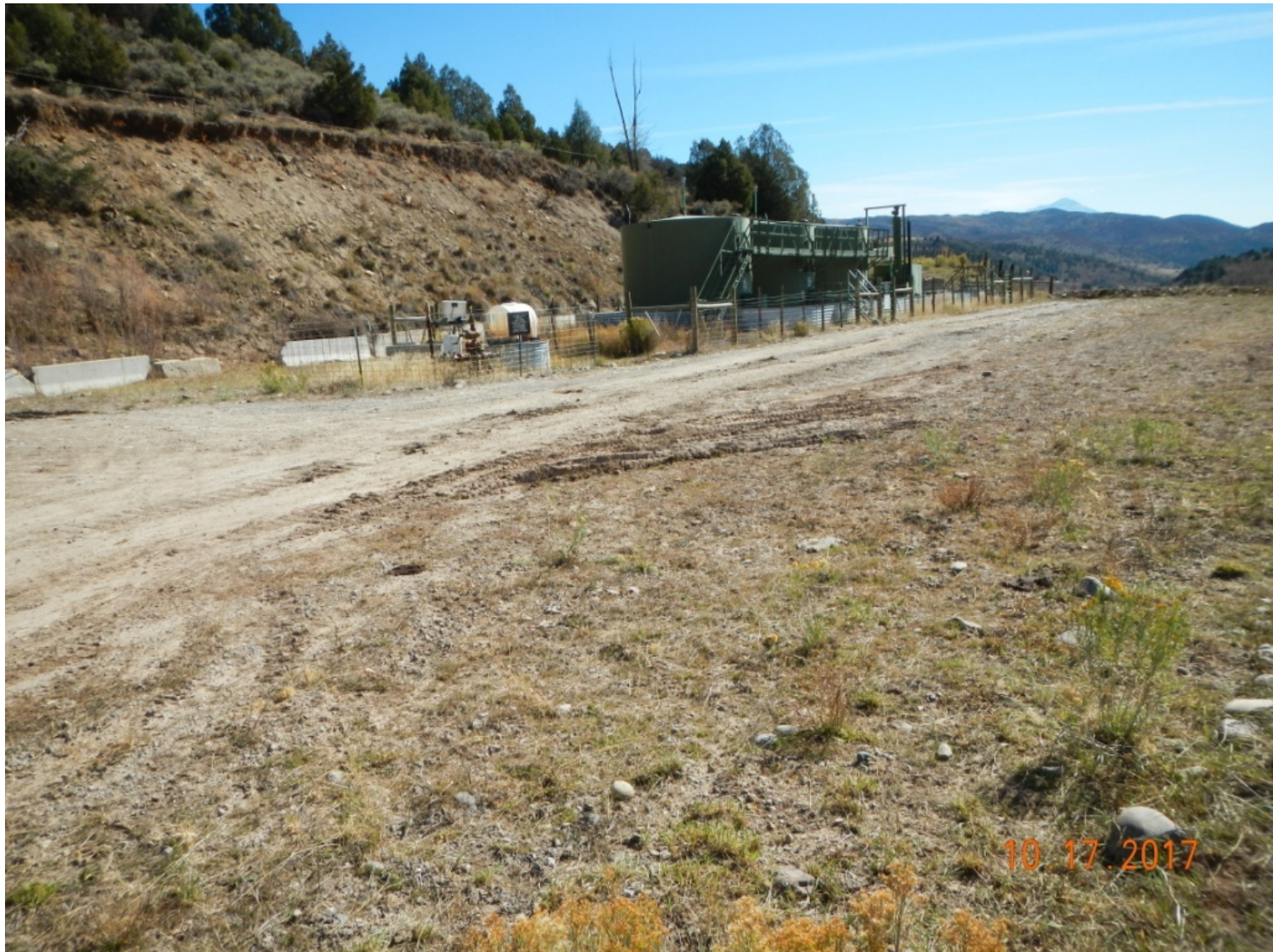
Photo 1. View of the project area from the northwestern corner of the working area facing center.
