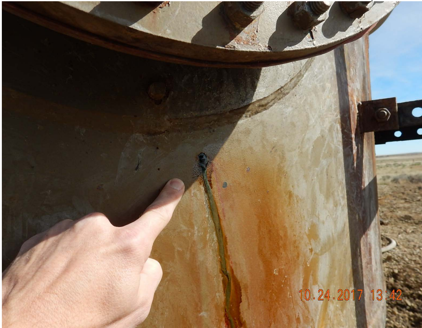
Small hole in heater treater was actively leaking during inspection.
