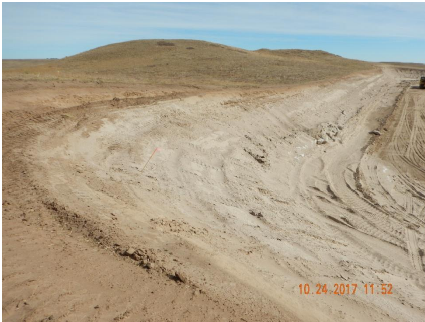
Photo 5. Photo taken from the northwest location, facing East. Operator shall control both run-off and run-on onto location. Operator shall stabilize all cut slopes to minimize site degradation.
