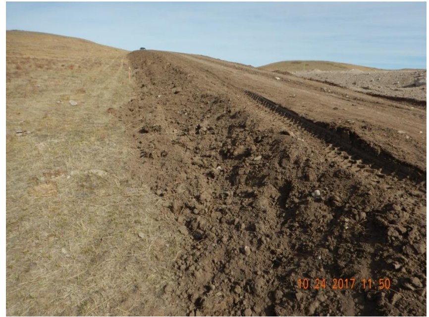
Photo 4. Photo taken from the western location, facing North. Appears topsoil has been salvaged and stored along the western perimeter of the location. No observed stormwater and erosion control BMPs around the topsoil stockpile.
