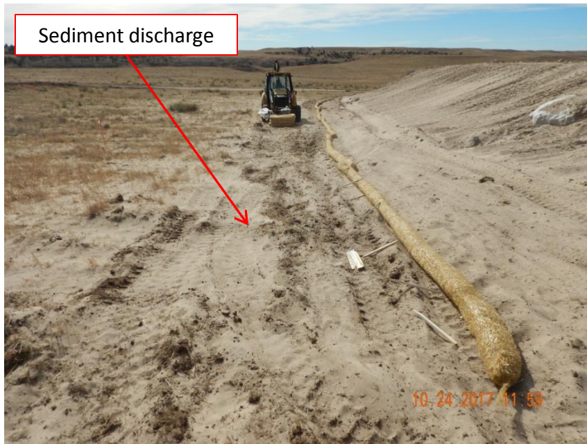
Photo 11. Photo taken from the eastern location on the fill slope, facing South. Operator starting to install straw wattle BMPs. Sediment discharge off location from wind erosion evident. Straw wattle BMPs are only temporary BMPs and should be used in conjunction with other BMPs.
