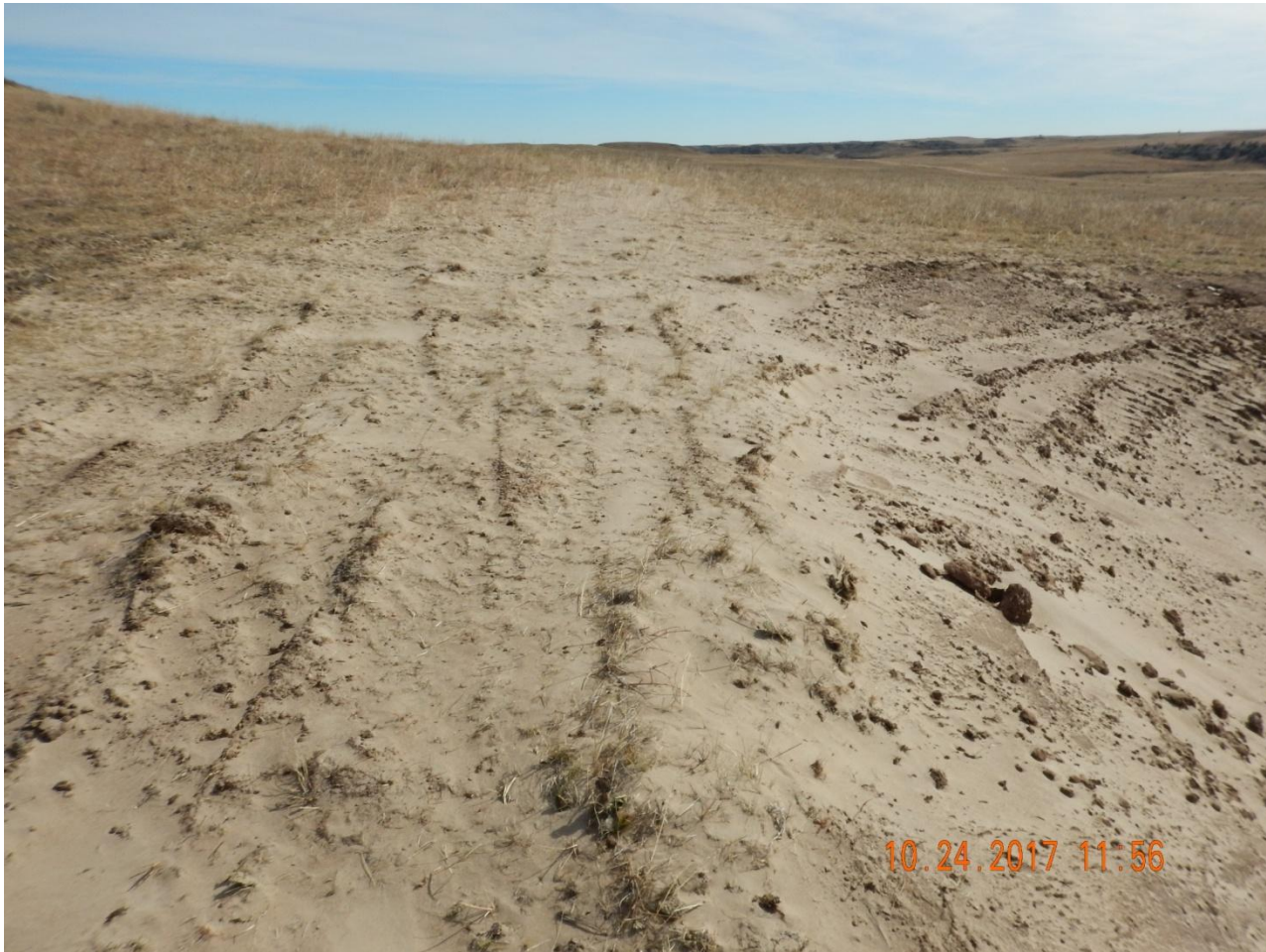
Photo 8. Photo taken from the northeast location, facing East. No observed stormwater and erosion control BMPs. Sediment discharge off location from wind erosion is evident along the northeast, east and southeast areas of the location.
