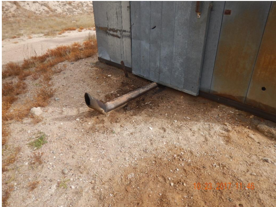
Photo 11: Photo taken from the west end of the pump unit. Photo shows dark discolored soil that can be found around the unit, as well as inside.
