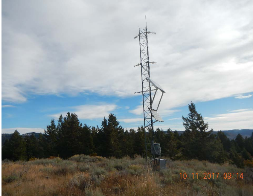
Communications tower looking SE
