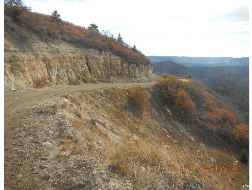
Access road looking NE
