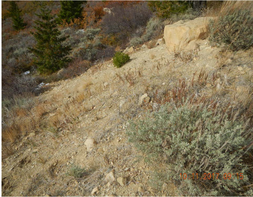
Fill slope south edge of pad
