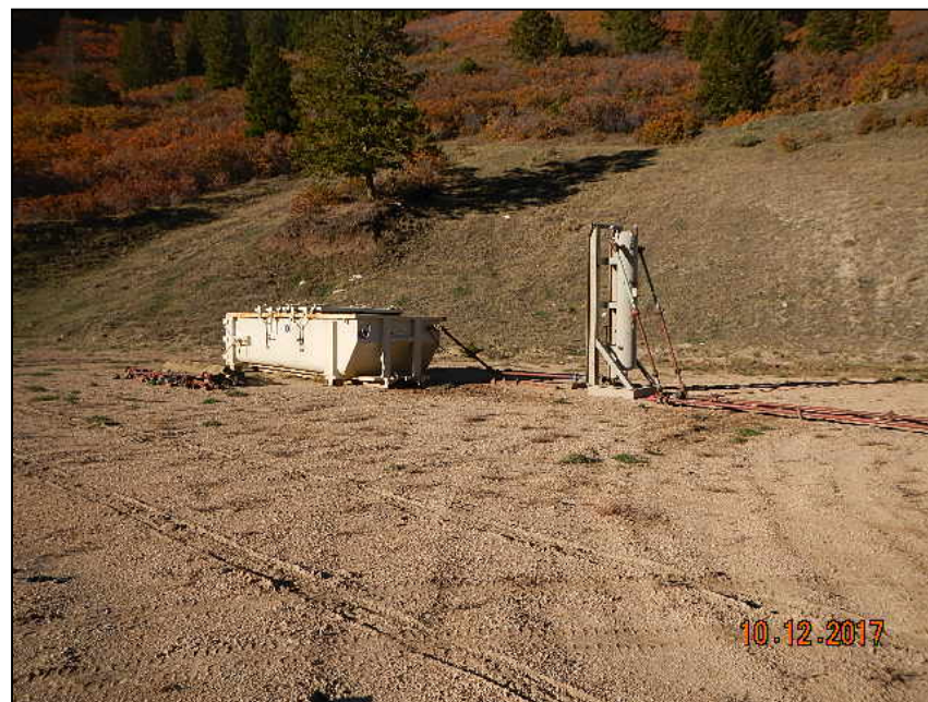
Photo 2. No containment around tank.
