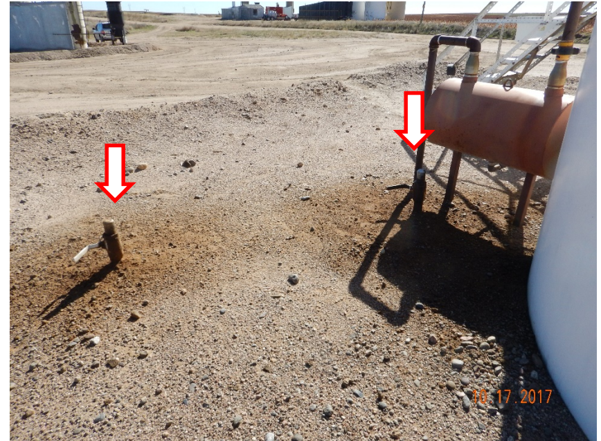
Photo #20 – Oil-stained soil and two bullplugged 2” steel flowline risers east of crude oil ASTs.
