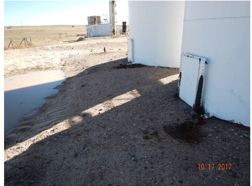
Photo #22 – Historical accumulation of oily waste beneath valves on north side of crude oil ASTs (1).
