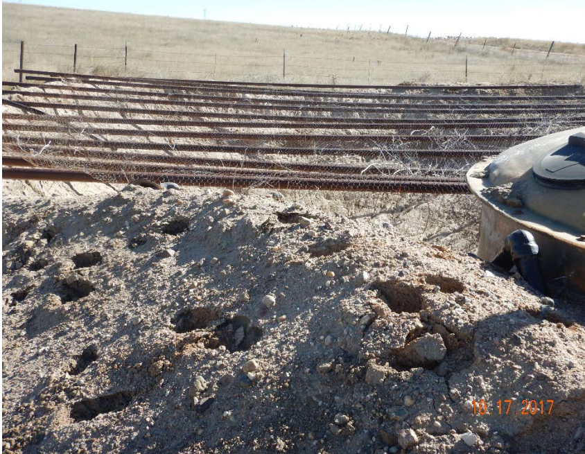
Photo #13 – Damaged pit berm at NW corner.
