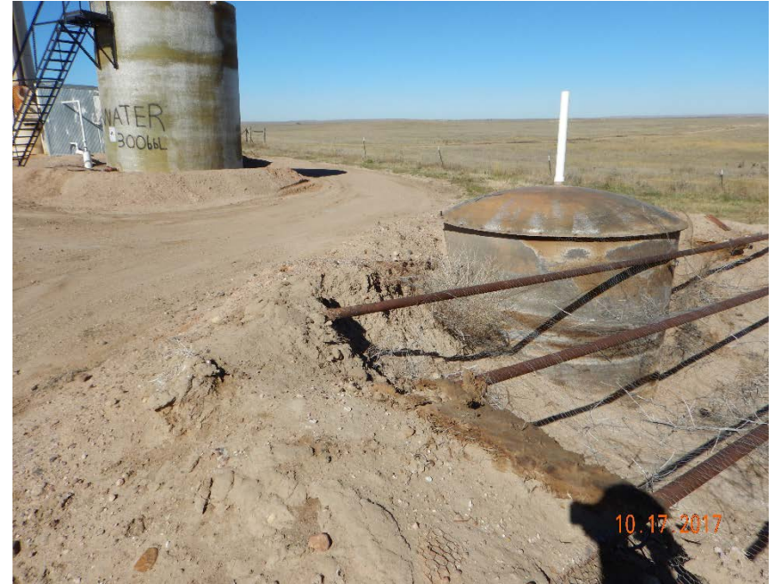
Photo #10 – Oil-stained soil at SW and NW corners of pit berm.
