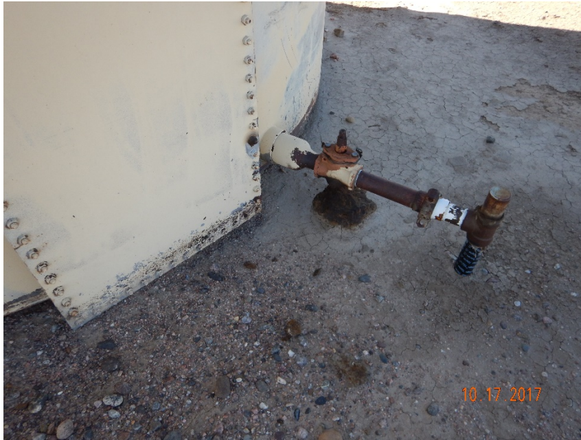
Photo #23 - Historical accumulation of oily waste beneath valves on north side of crude oil ASTs (2).
