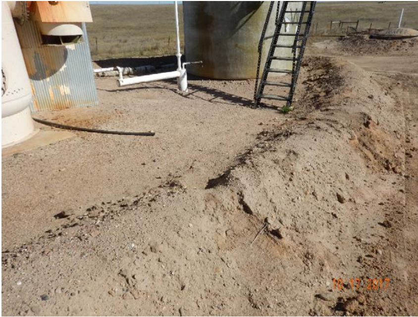
Photo #15 – Earthen berm for produced water tank is shallow, damaged, and eroded. View of SE corner.
