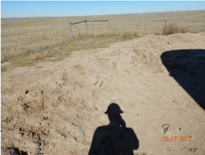
Photo #25 - Damaged and eroded portion of earthen berm NW of crude oil ASTs.
