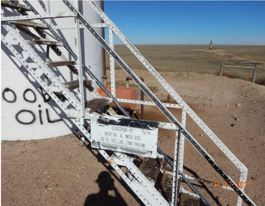
Photo #19 – Battery sign located at SE corner of crude oil tank battery. Operator’s contact information decal is flaking off of sign, rendering emergency contact phone number illegible.
