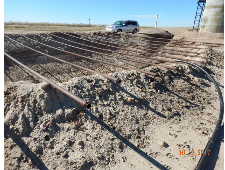
Photo #8 – Pit berm is damaged and eroded on all sides (view from NE corner).
