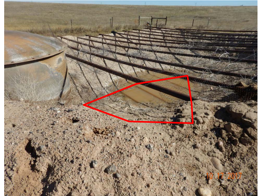
Photo #12 – Additional photo of large gaps in wildlife cover.
