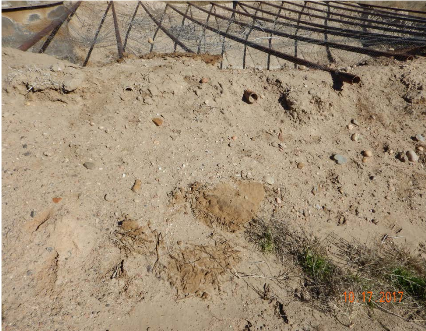
Photo #11 – Oil stained soil outside of pit berm at SW corner.
