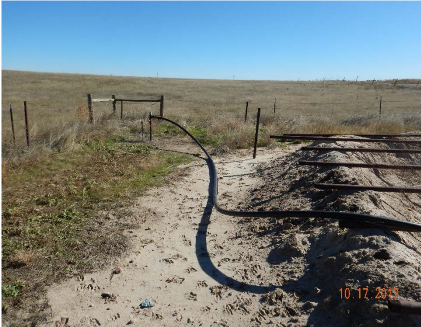
Photo #7 – 2" Flowline riser NE of produced water pit is plumbed to discharge into pit. Note: 1" flowline riser north of 2" and wildlife tracks in sediment north of pit berm.
