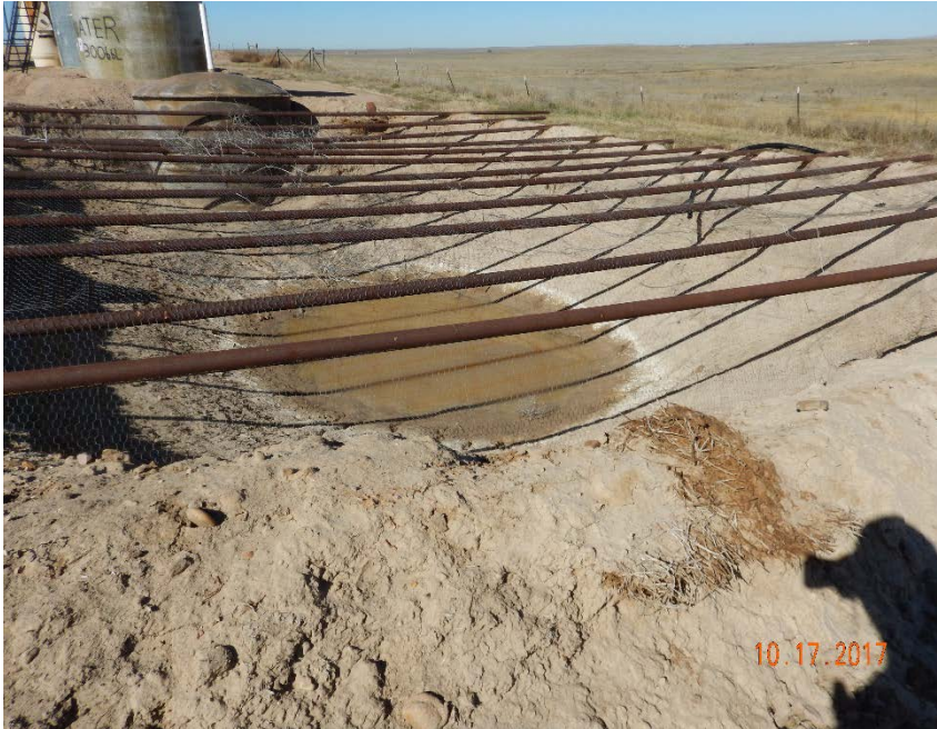
Photo #9 – Localized, oil-stained soil with vegetation incorporated into east pit berm.
