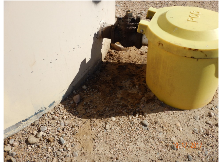
Photo #24 - Historical accumulation of oily waste beneath loadout valve on south side of crude oil AST.
