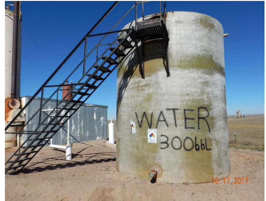
Photo #14 – 300 bbl fiberglass produced water AST shares shallow earthen berm with separator shed.
