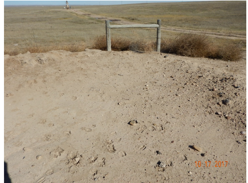
Photo #26 – Shallow, eroded portion of earthen berm NE of crude oil ASTs.
