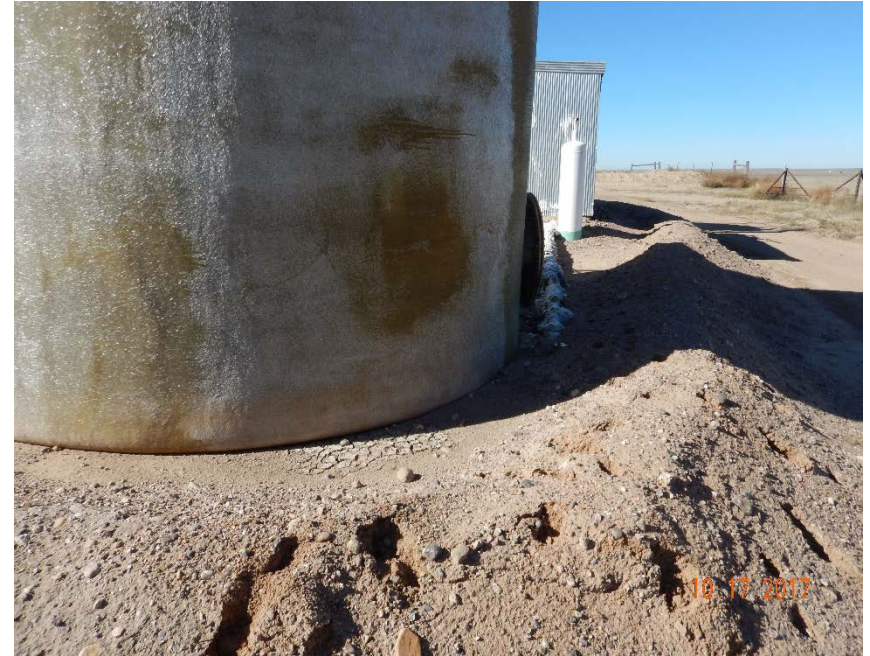
Photo #16 – View of damaged, shallow earthen berm at NE corner of produced water AST. Berm footprint is of insufficient size to satisfy Rule 605.a.(4).
