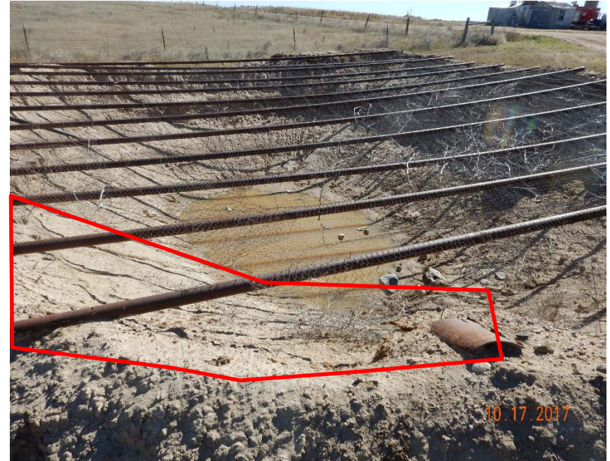
Photo #6 – Gaps in mesh around produced water pit are large enough to allow wildlife access.
