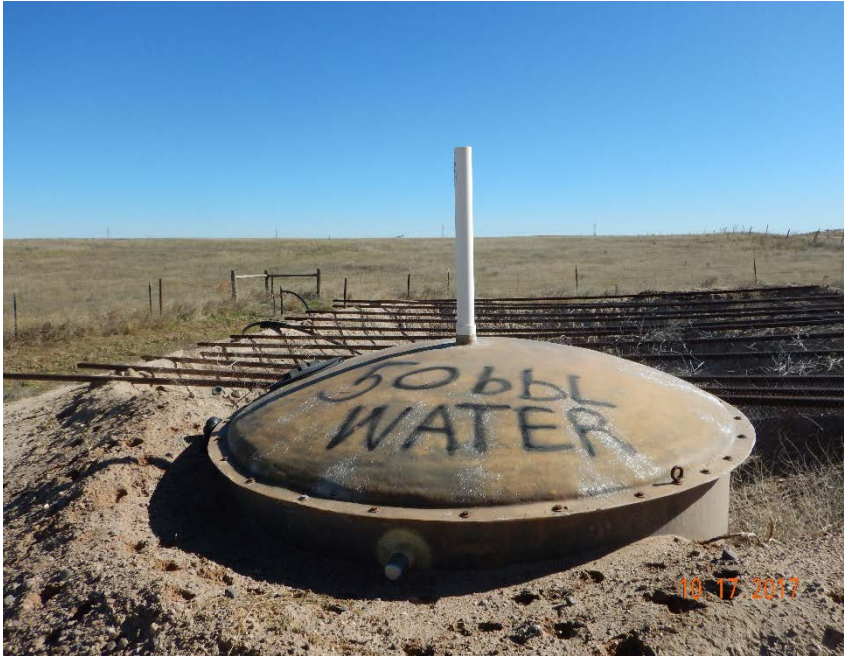
Photo #5 – View of 50 bbl skim tank and produced water pit from west side. Note: skim tank lacks NFPA placard.
