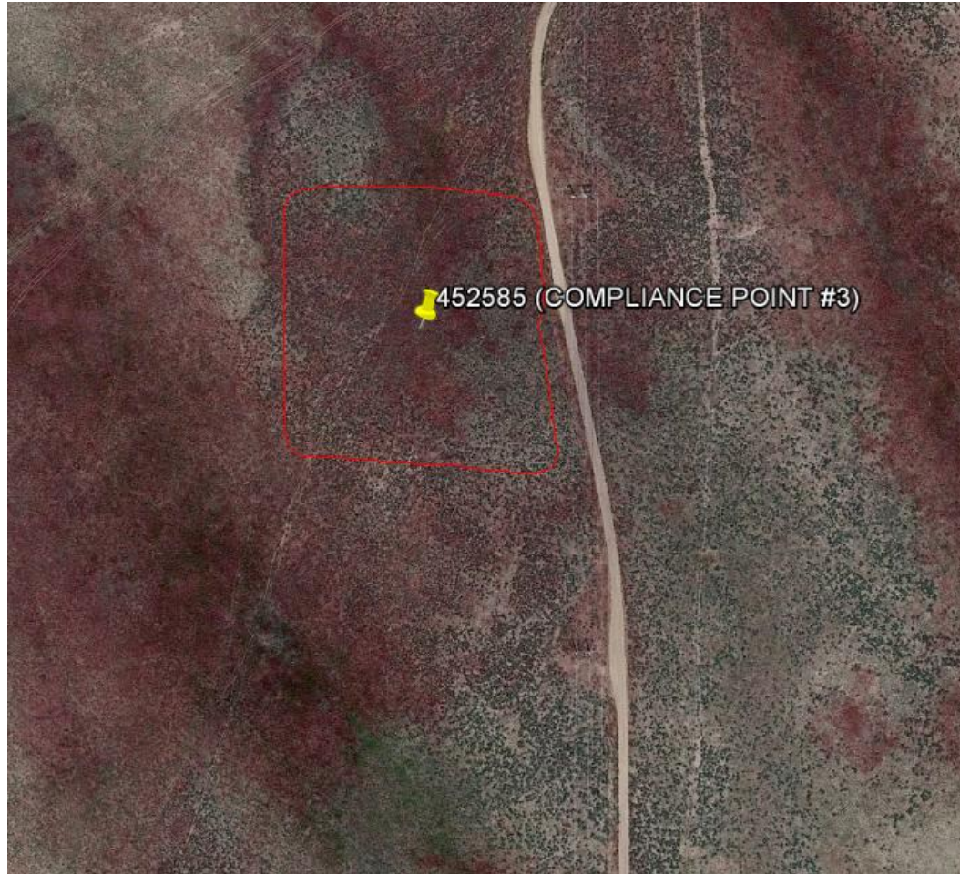
Photo 1. Google Earth aerial imagery taken on June 14, 2016. Operator has constructed a pad in the northeast of Section 34, Township 4N, Range 63W without an approved 2A- see Photo 2. The approximate center of the pad is at the following Latitude/Longitude: 40.271549/-104.416259. A disturbance area of 4.47 acres was mapped on 10/12/2017 using a Trimble Juno 3B handheld device (red line).
