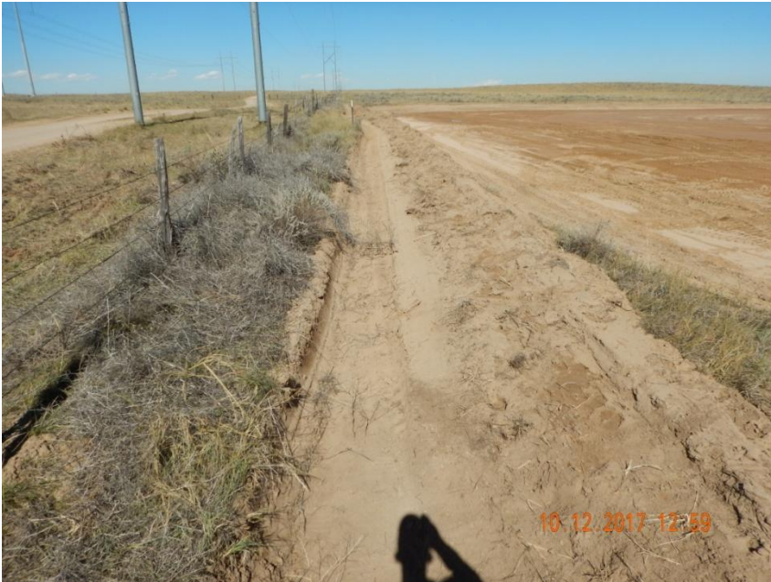
Photo 3. Photo taken from the western location, facing North. Operator has installed a ditch and berm around the entire location perimeter. The berm BMP has been left unconsolidated which would not be considered in proper functioning condition.
