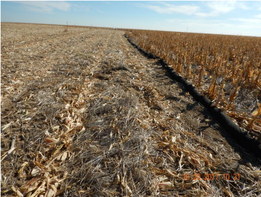
Photo 3. Photo taken from the southern location, facing East. Operator has cut/mowed disturbance area and has installed a temporary BMP (i.e., filtrex wattle) around the entire perimeter of the location.
