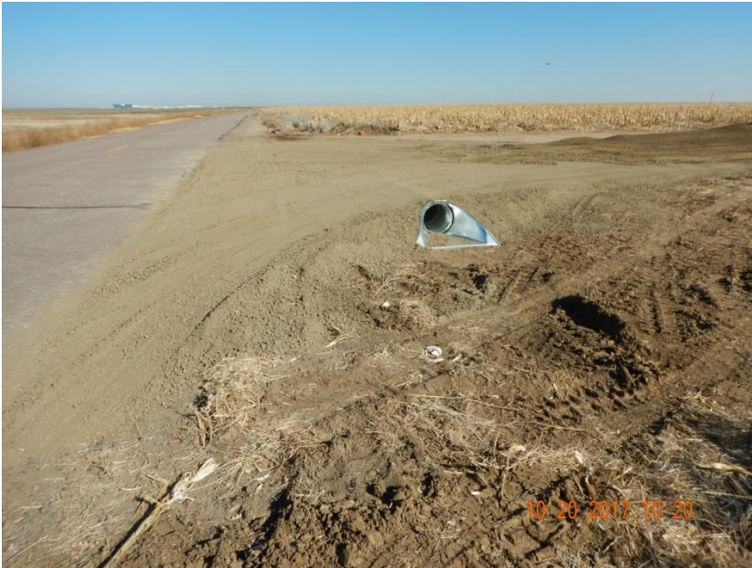
Photo 1. Photo taken from the entrance of location, facing North. Operator constructing approach for the entrance of location. Culvert has been installed in conjunction with gravel.
