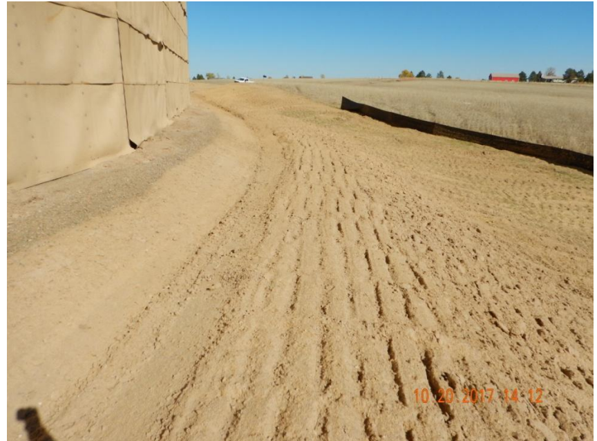
Photo 8. Photo taken from the southern location, facing East. Ditch BMP has been installed that is directed to a retention pond area with silt fence BMP downgradient. Appears fill slope areas have been temporarily stabilized with hydromulch and tracked with equipment.
