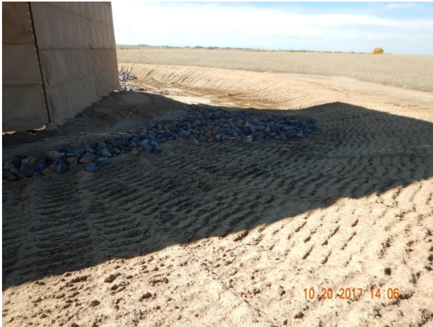
Photo 3. Photo taken from the northeast location, facing West. Retention pond has been installed with inlet protection devices (rip-rap). Perimeter disturbance areas have been temporarily stabilized with hydromulch and tracked with equipment.
