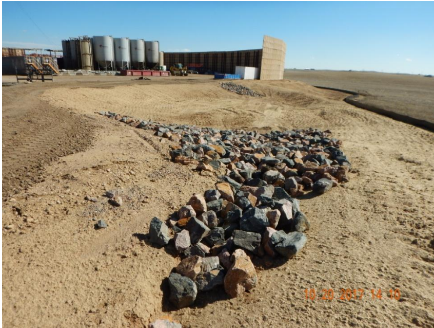
Photo 7. Photo taken from the western location, facing South. Retention pond has been installed with inlet protection devices (rip-rap). Silt fence BMP has been installed along the southwest and southern location perimeter. Disturbance areas have been temporarily stabilized with hydromulch and tracked with equipment.
