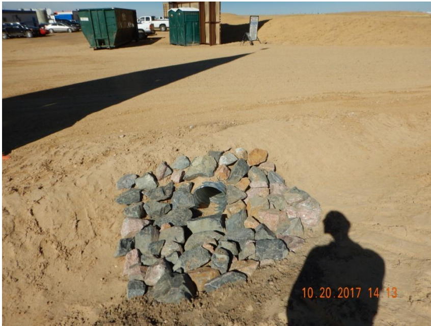
Photo 9. Photo taken from the entrance of the location, facing North. Inlet and outlet devices (rip-rap) have been installed in conjunction with the culvert.
