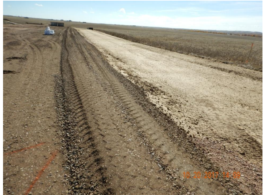
Photo 6. Photo taken from the northwestern location, facing South. Operator has installed a berm BMP using compacted gravel. Western outer perimeter disturbance area has been temporarily stabilized with hydromulch.
