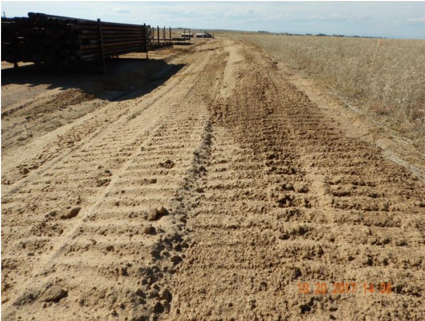
Photo 5. Photo taken from the northern location, facing West. Ditch BMP has been installed that is directed to a retention pond area. Perimeter disturbance areas have been temporarily stabilized with hydromulch and tracked with equipment.
