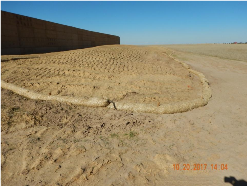
Photo 1. Photo taken from the entrance of location, facing North. 2 Topsoil stockpiles are located along the eastern location. Appears topsoil stockpiles have been hydromulched and tracked with equipment. Straw wattles have been installed around the topsoil piles.
