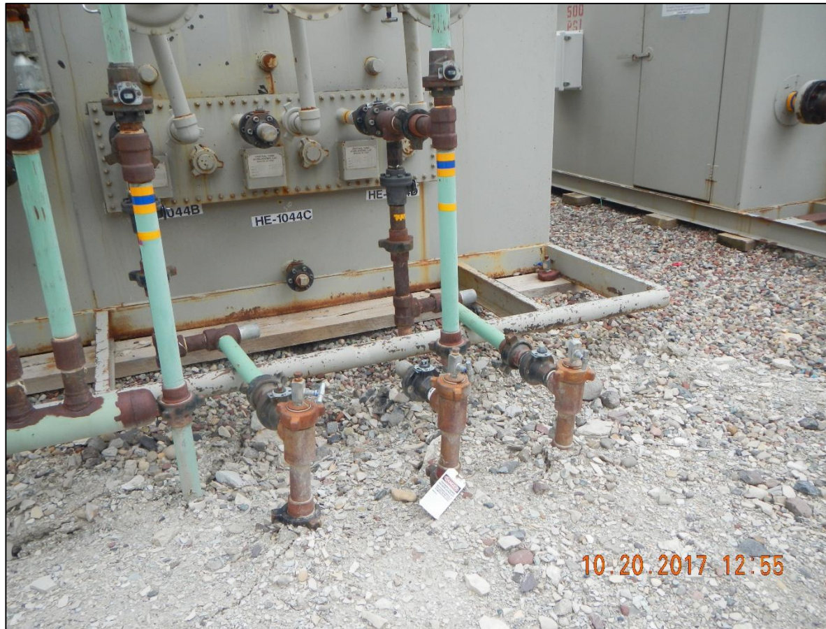
Unused 2" riser with plug cap and Lock out tag.
