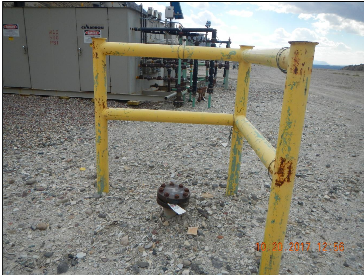
Unused 4" riser with plug cap and Lock out tag.
