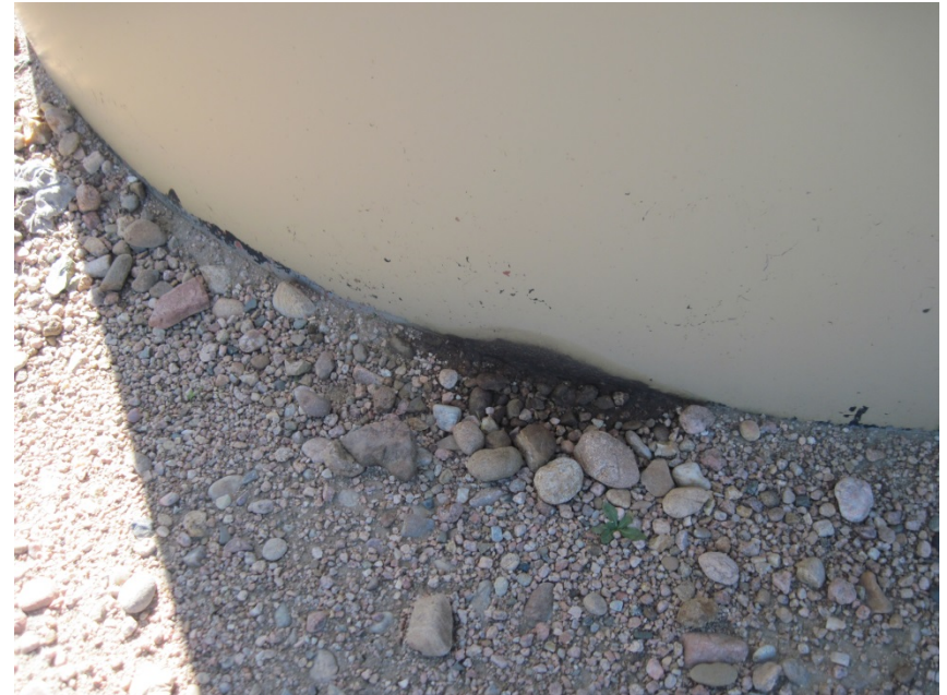
HOLE IN WEST PROD OIL TANK AND SOILED DIRT AROUND HOLE
