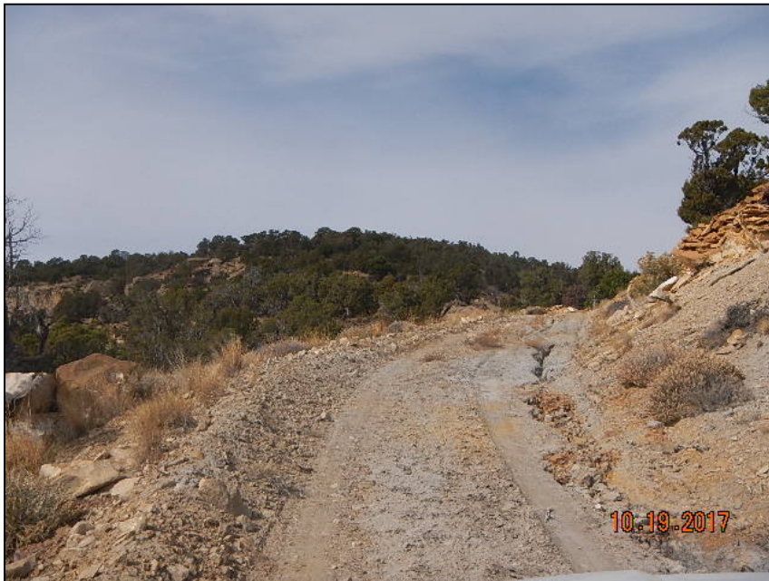
Photo 1. Main road to location has multiple areas of erosion across roadway and sediment migration down gradient of road surface.
