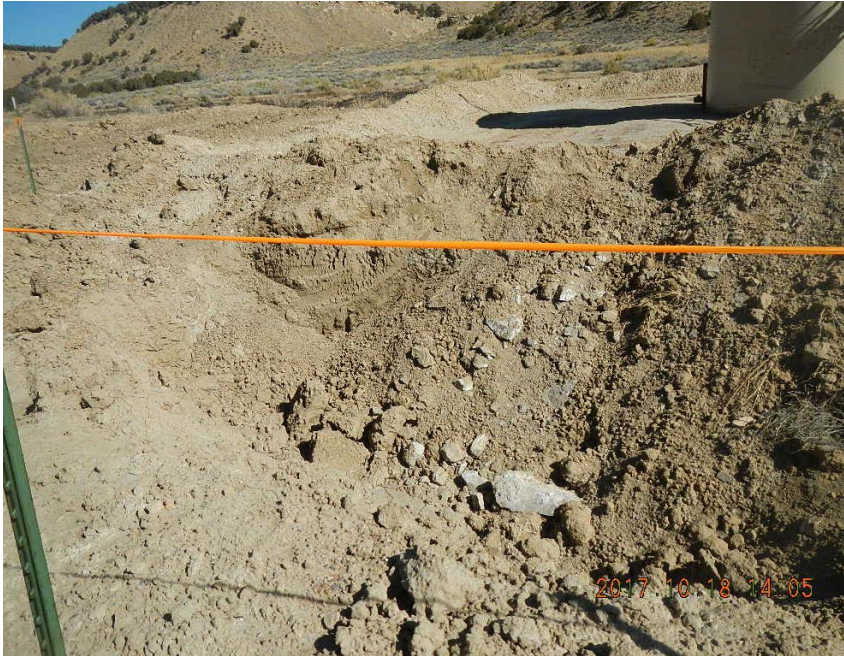
An approximate 30' x 10' x 15' deep excavation.
