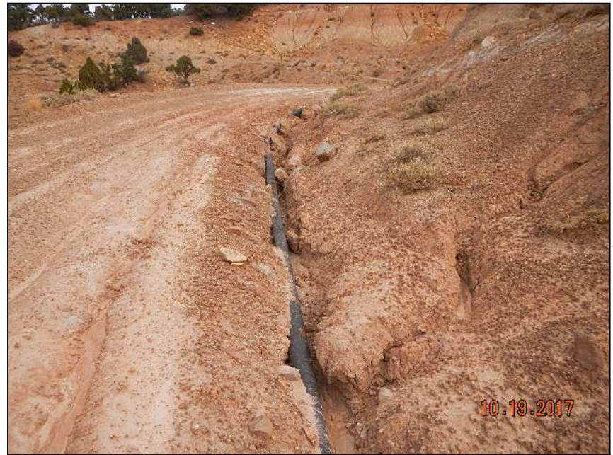
Photo 2. Exposed pipeline in roadway.
