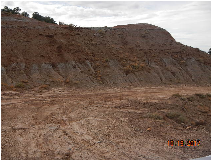
Photo 1. Access road to location has multiple areas of erosion and sediment migration down gradient of road surface.
