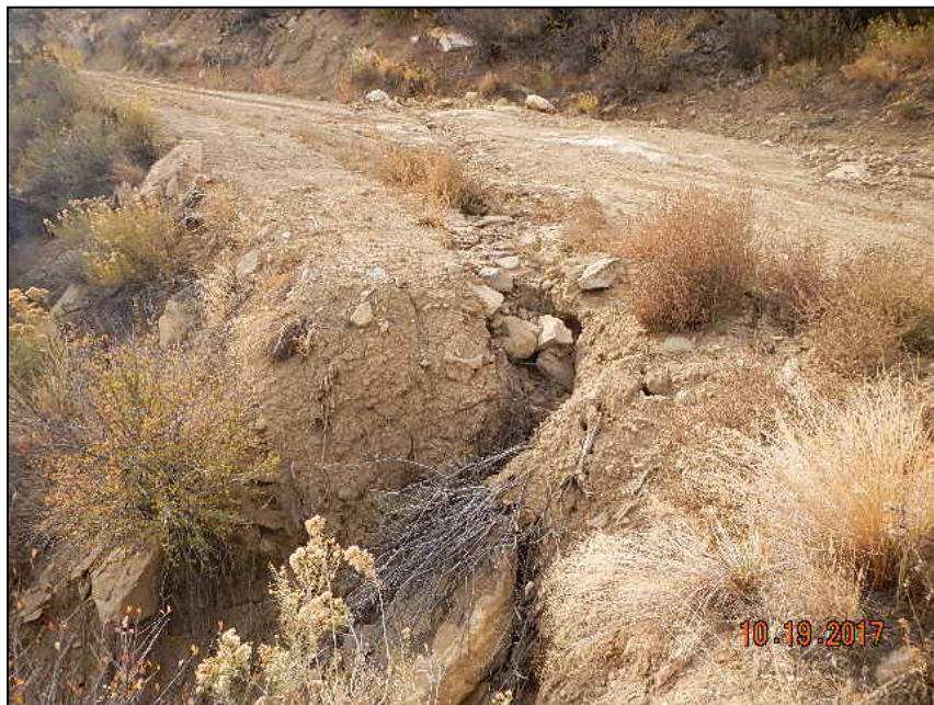
Photo 3. Main road from Baxter Pass Road to location has multiple areas of erosion and sediment migration down gradient of road surface
