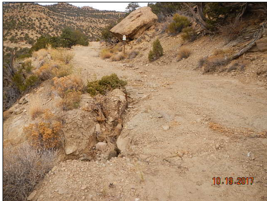
Photo 4. Main road from Baxter Pass Road to location has multiple areas of erosion and sediment migration down gradient of road surface
