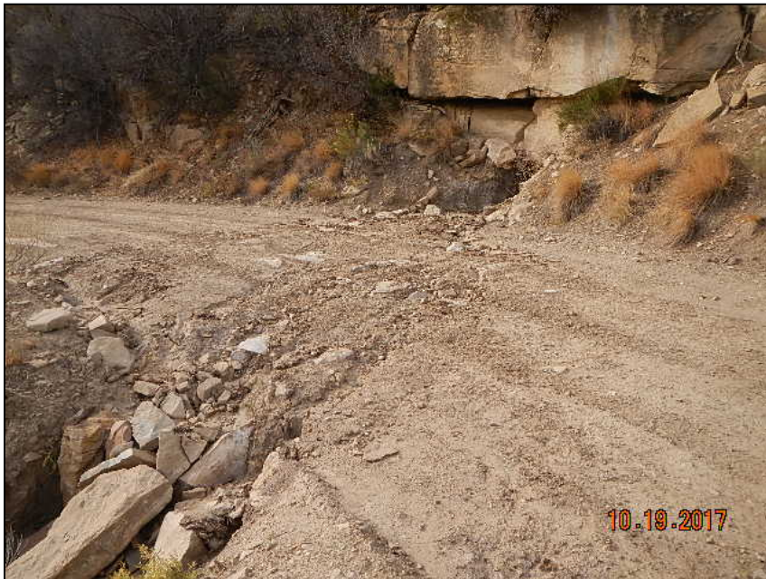
Photo 1. Main road from Baxter Pass Road to location has multiple areas of erosion and sediment migration down gradient of road surface.
