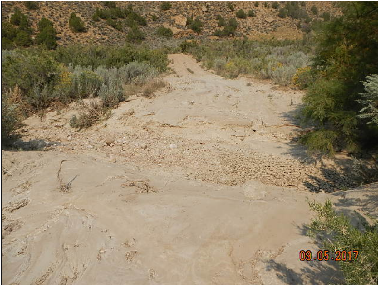
Photo 1. Access road has been washed out. No access to location at time of inspection.
