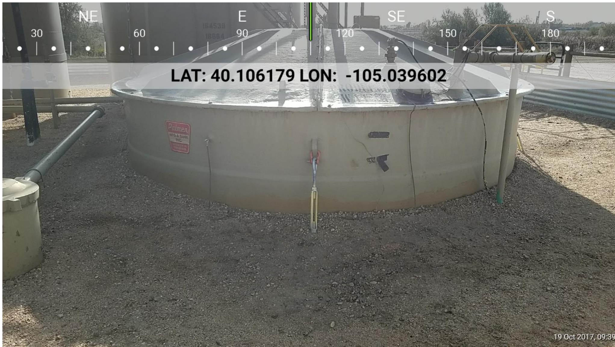
Flood Anchor on Produced Water Tank
