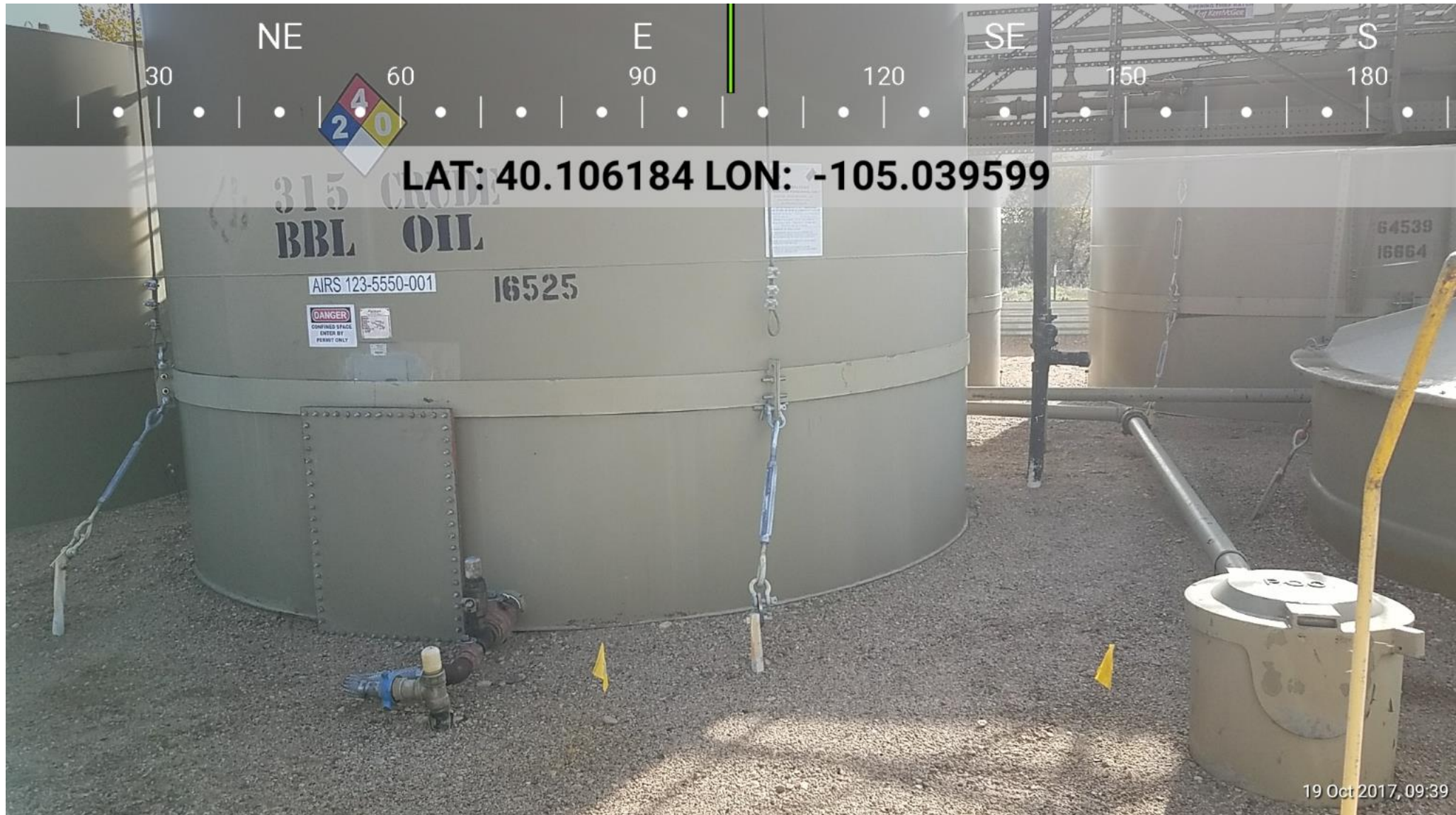
Flood Anchor on Crude Oil Tank
