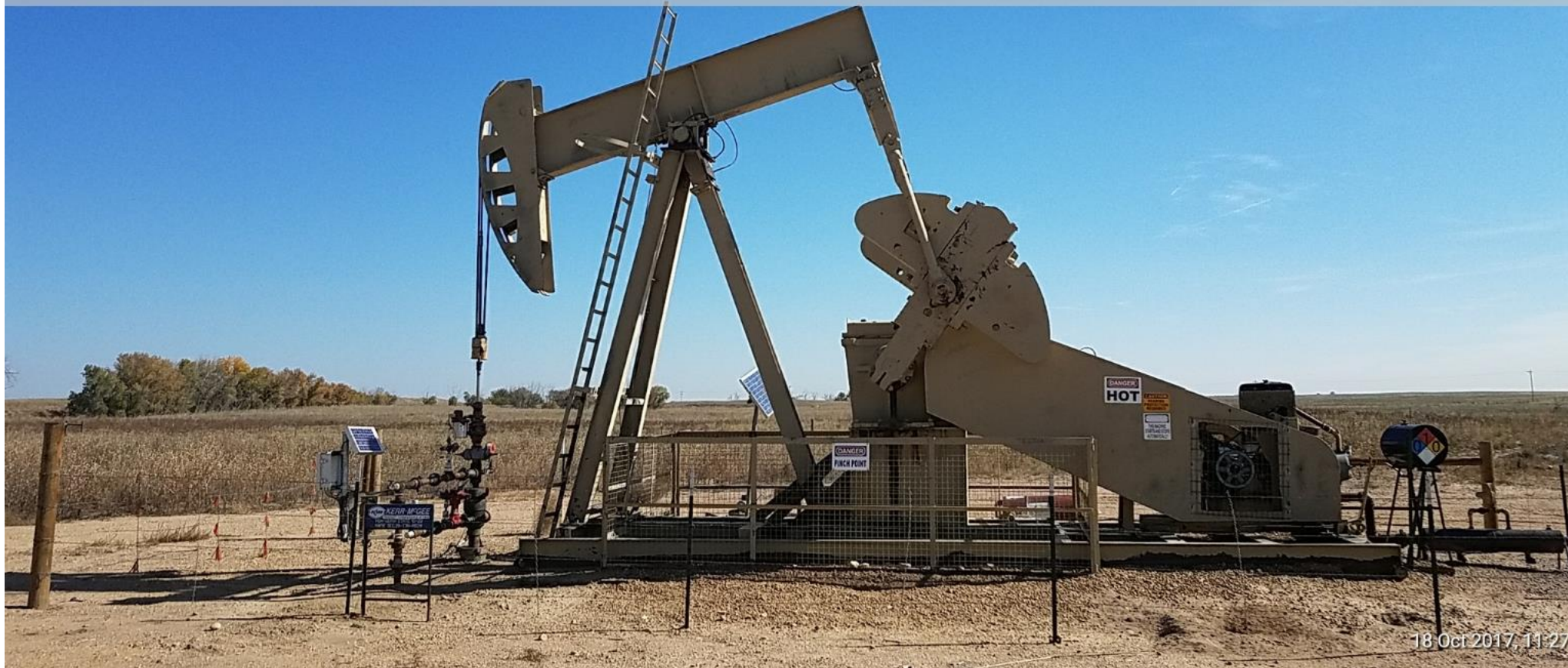
Pump Jack Location Number: 330530
