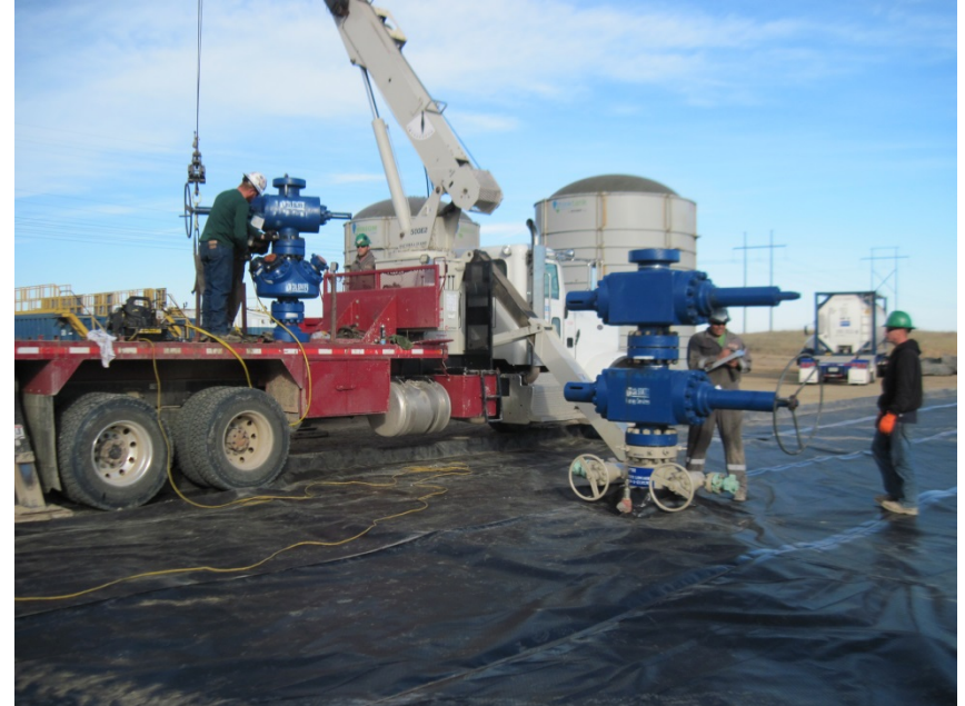
PUTTING GOAT HEAD ON WELLHEAD
