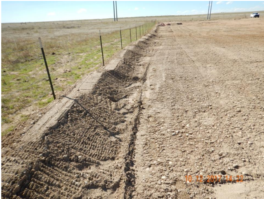
Photo 3. Photo taken from the eastern location, facing South. Appears the Operator has installed a berm BMP. The berm BMP appears sufficiently compacted but shall be monitored to ensure compaction holds up overtime.
