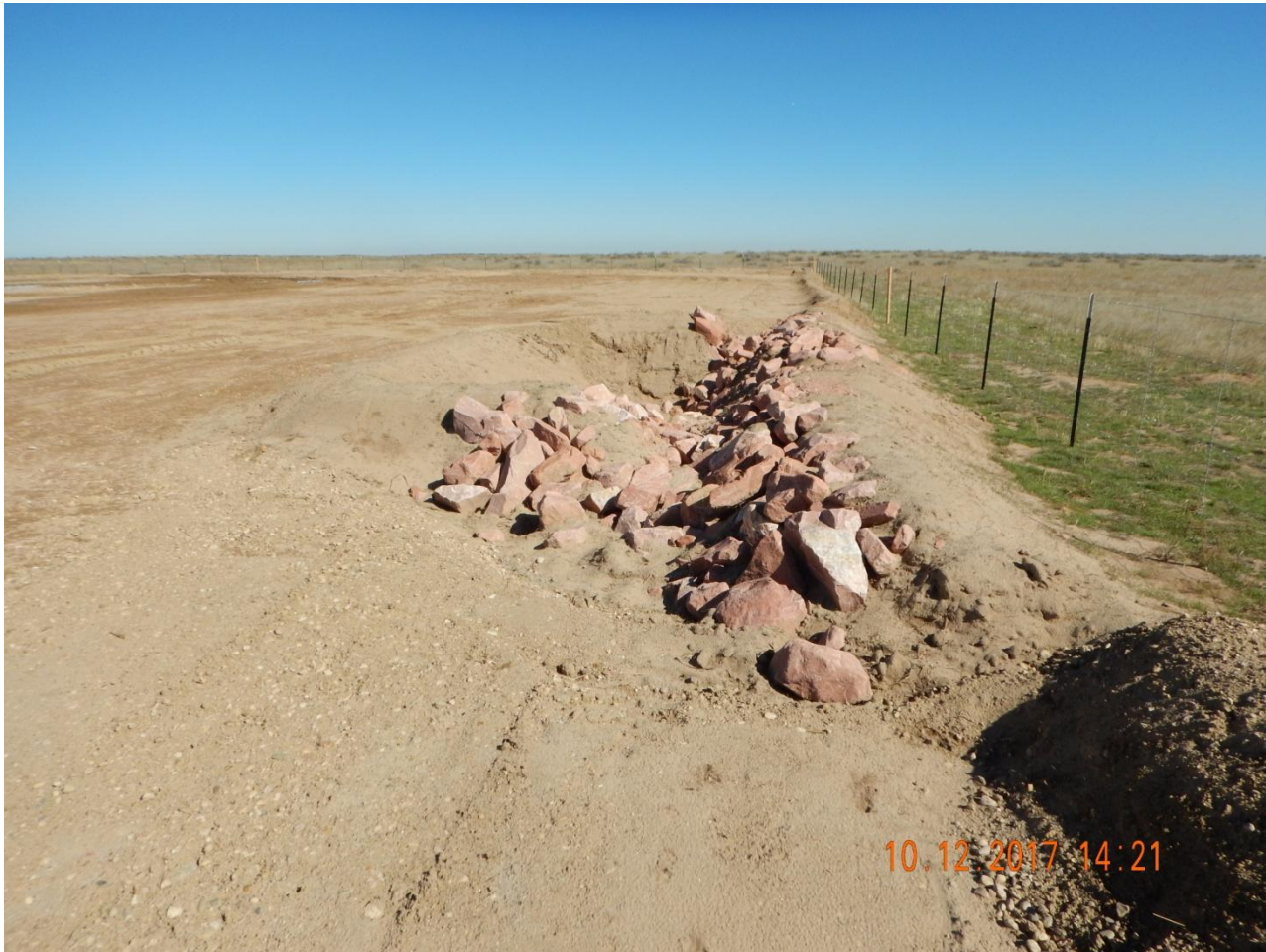
Photo 2. Photo taken from the southern location, facing East. Appears the Operator has installed a sediment trap with both inlet and outlet devices.
