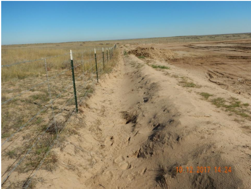
Photo 5. Photo taken from the western location, facing North. Appears the Operator has installed a ditch and berm BMP. Berm BMP appears to be left unconsolidated. Operator shall monitor BMP as this could be susceptible to wind and water erosion overtime.
