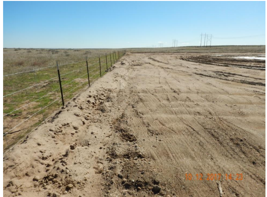
Photo 4. Photo taken from the northern location, facing East. Appears the Operator has installed a berm BMP but has been left unconsolidated.
