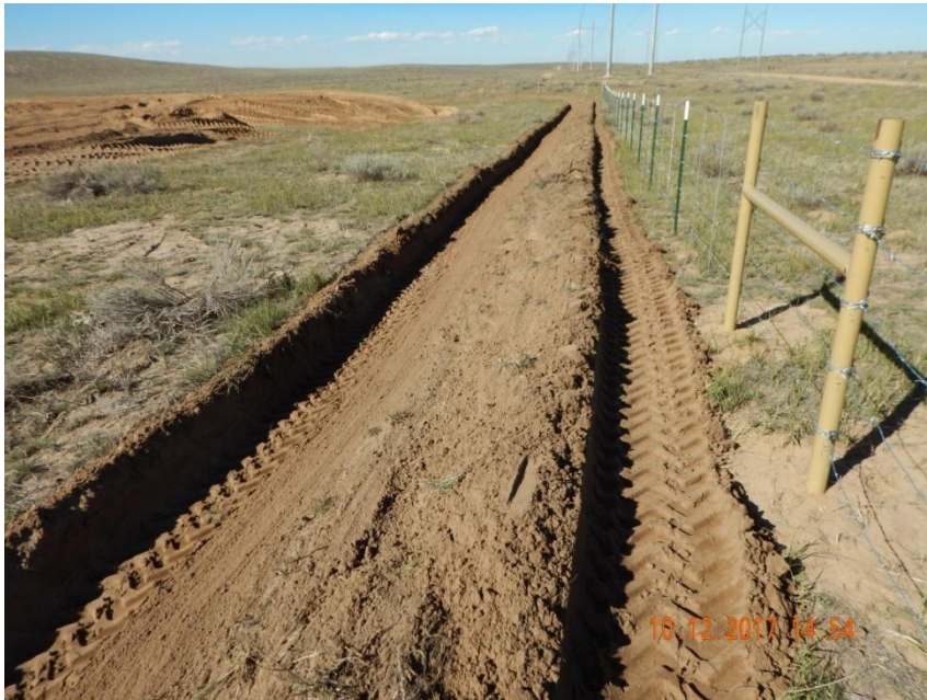
Photo 8. Photo taken from the eastern location, facing South. Operator installed a ditch and berm BMP after COGCC staff communicated to the Operator stormwater management requirements. The berm BMP has not been properly compacted and left unconsolidated.
