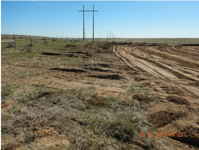
Photo 2. Photo taken from the eastern location, facing South. Operator has failed to install stormwater and erosion control BMPs prior to, or at, the beginning of construction.
