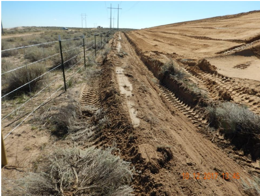
Photo 2. Photo taken from the eastern location, facing South. Operator has installed a ditch and berm around the entire location perimeter. Portions of the berm BMP have not been properly compacted and have been left unconsolidated.
