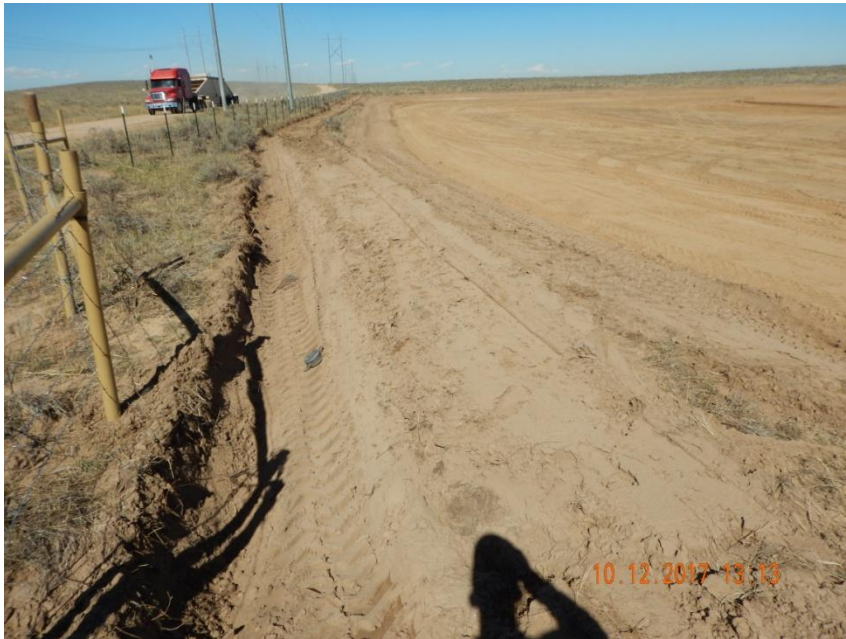
Photo 2. Photo taken from the western location, facing North. Operator has installed a ditch and berm around the entire location perimeter. Portions of the berm BMP have not been properly compacted and have been left unconsolidated.
