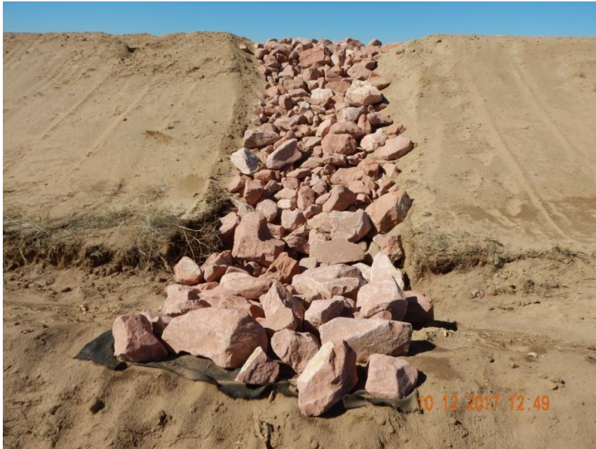
Photo 6. Photo taken from the eastern location, facing West. Operator has installed an armored ditch.
