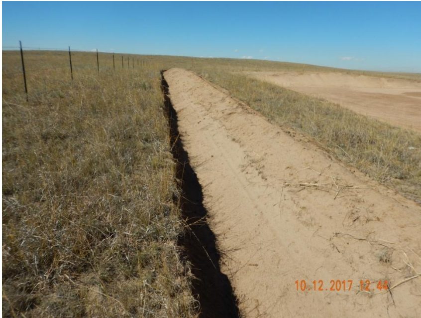
Photo 2. Photo taken from the southern location, facing West. Operator has installed a ditch and berm around the entire location perimeter.
