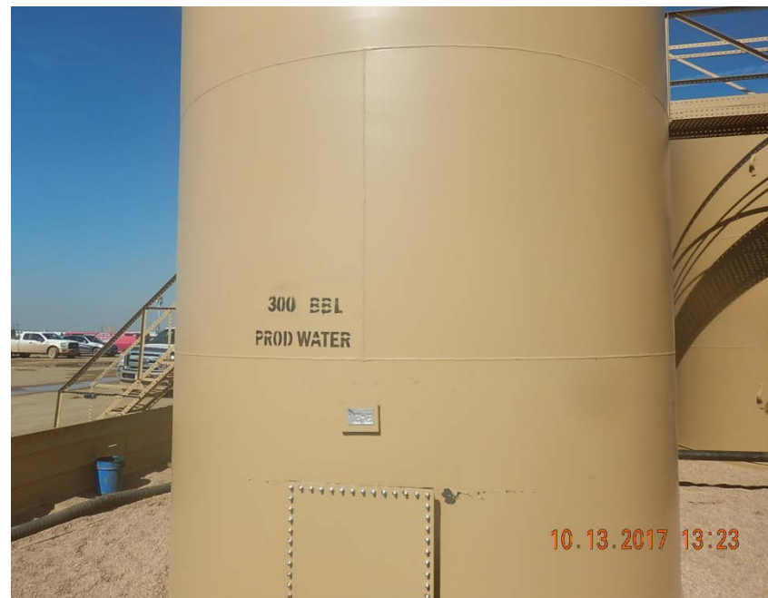
Photo 3: No decal on produced water tank
