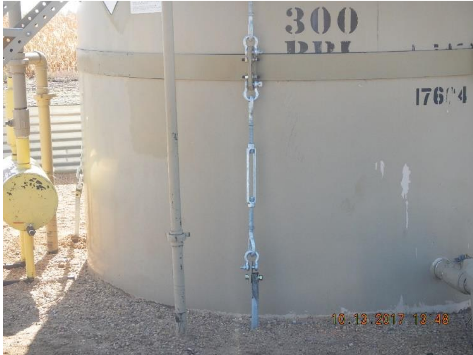
Flood Anchor on Crude Oil Tank
