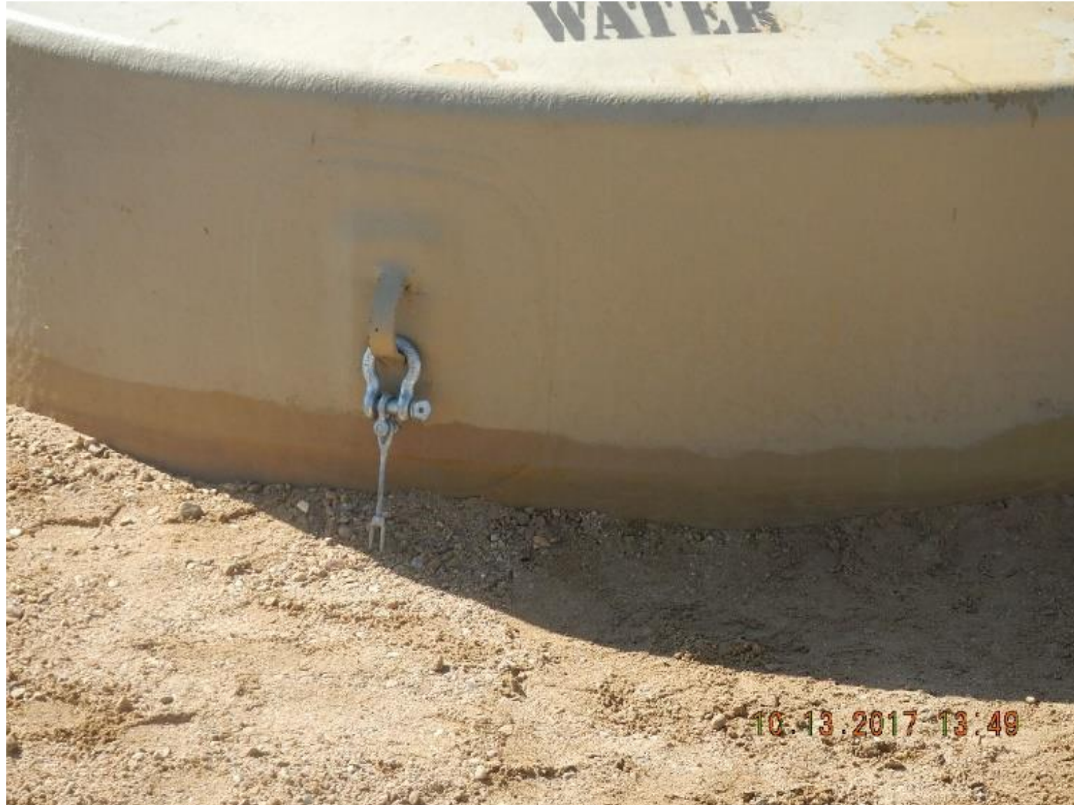
Produced Water Tank Flood Anchor
