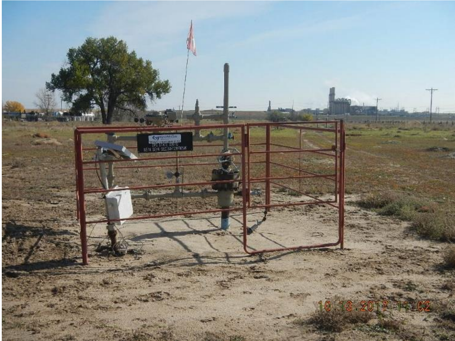
Wellhead from west Location Number: 310762
