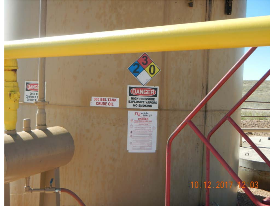
Crude oil tank placards
