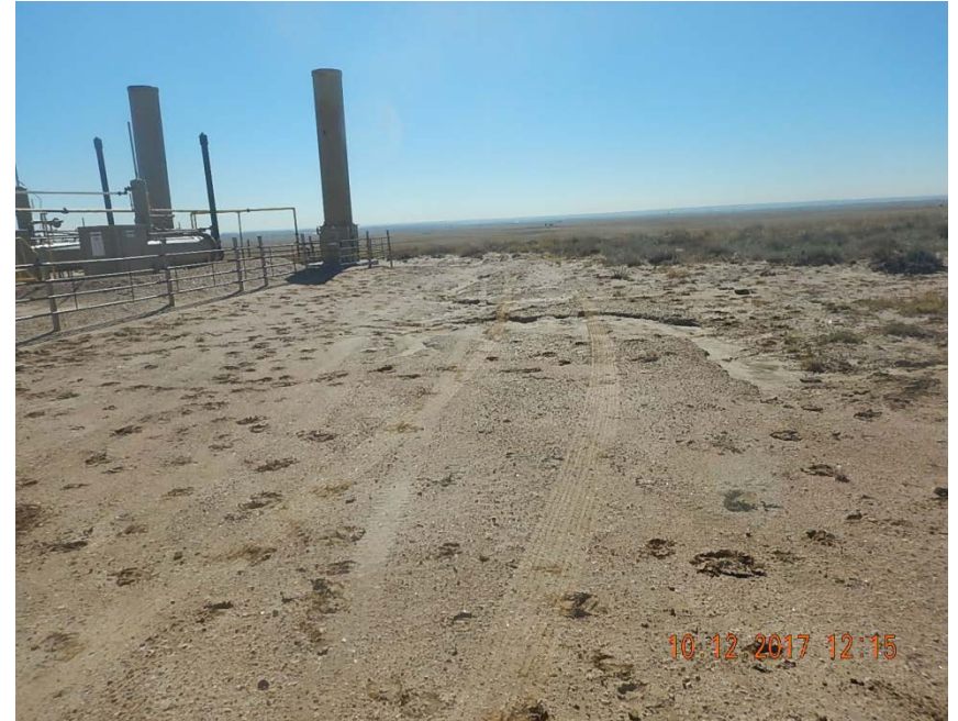
Photo 4: Stormwater erosion on SW corner of location
