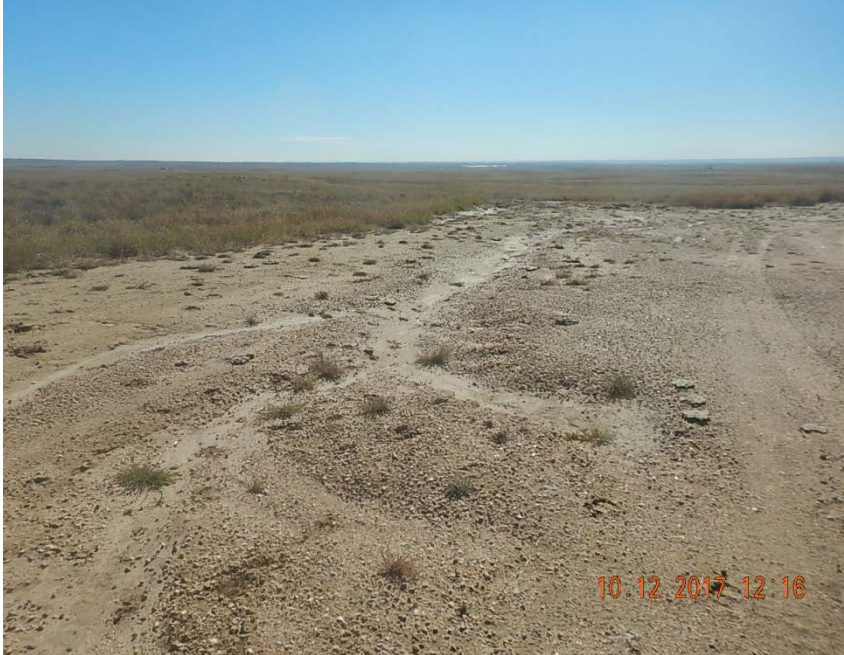
Photo 5: Stormwater erosion on E side of location
