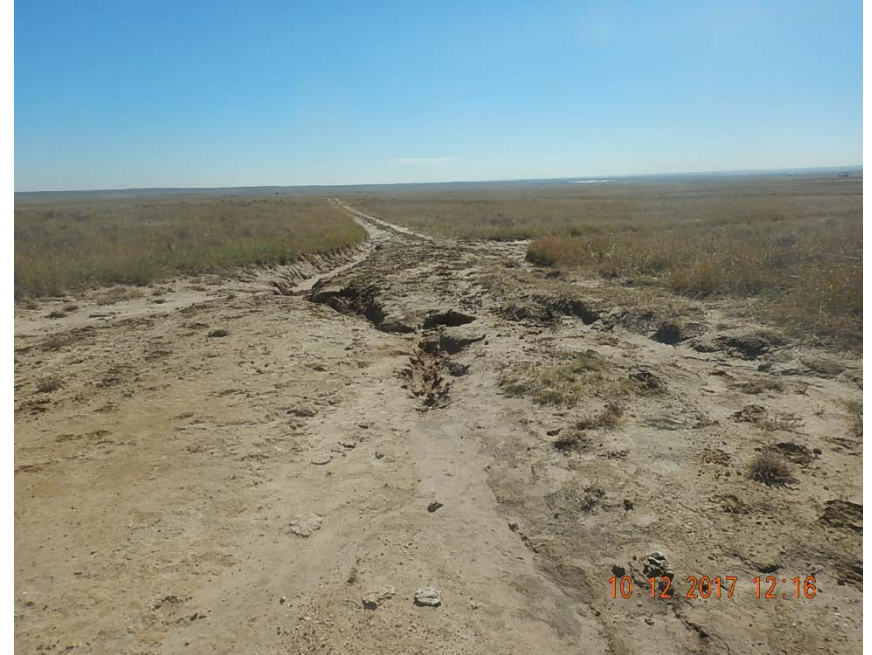
Photo 6: Stormwater erosion on SE side of location
