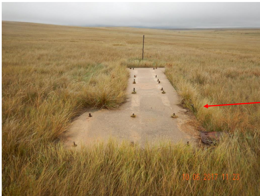
Photo 3: Photo taken from the north side of the well, facing south. Photo shows concrete pump base and pipe remaining on the location. This needs to be removed. Located ~ 39°54'31.87"N, 103°42'13.13"W
