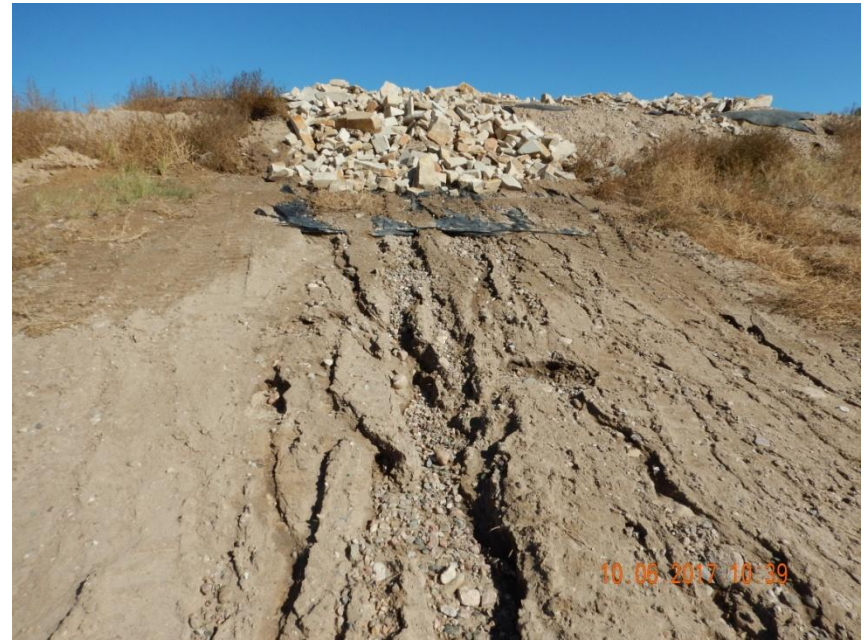
Photo 4. Photo taken from the southwestern location, facing North. Rill erosion forming into gully erosion observed down slope of the installed rock material.
