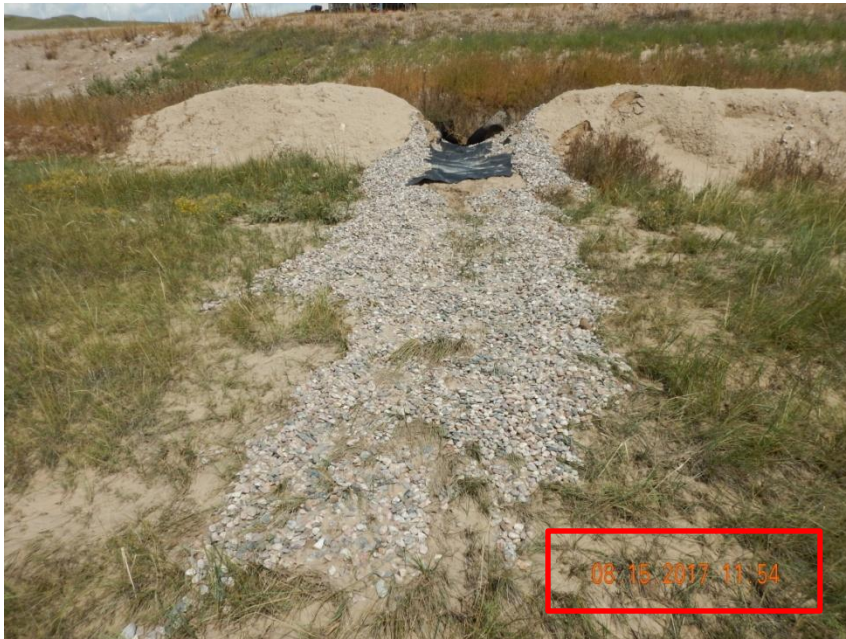
Photo 13. Photo taken on August 15, 2017 from the southeast sediment trap outlet area, facing North. Sediment trap does not appear to have a sufficient stabilized outlet. Rock material does not appear to be the appropriate size and the plastic-like material only appears to allow stormwater flows to accelerate out of the sediment trap.
