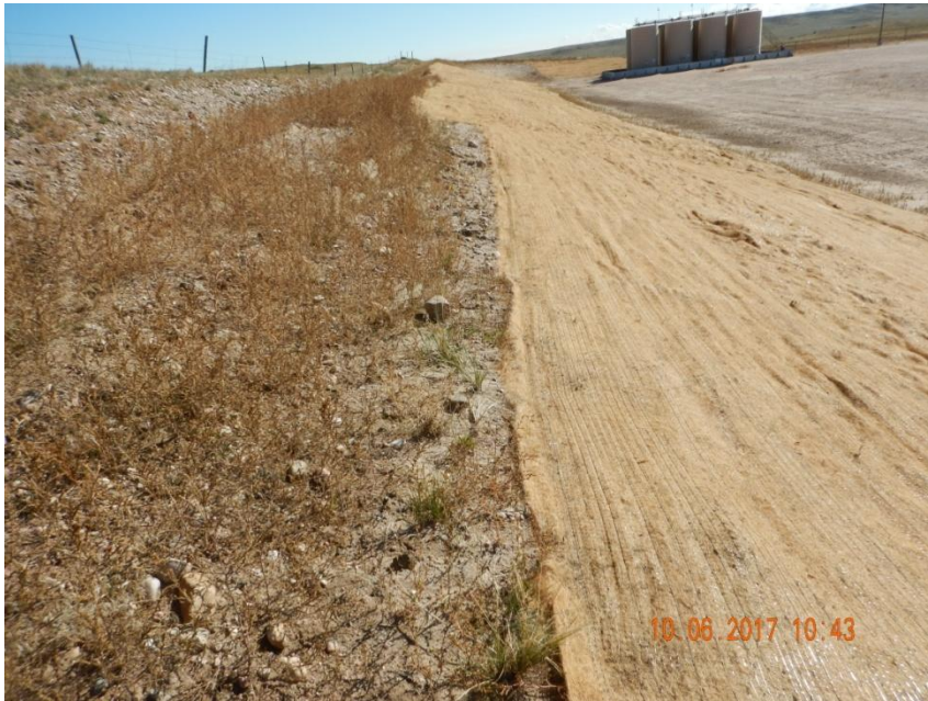
Photo 9. Photo taken from the northwestern cut slope area, facing East. Operator has not properly installed the erosion blanket using good engineering practices. Operator has not properly trenched and anchored BMP. Operator has not installed the BMP with good contact with the ground to avoid tenting.
