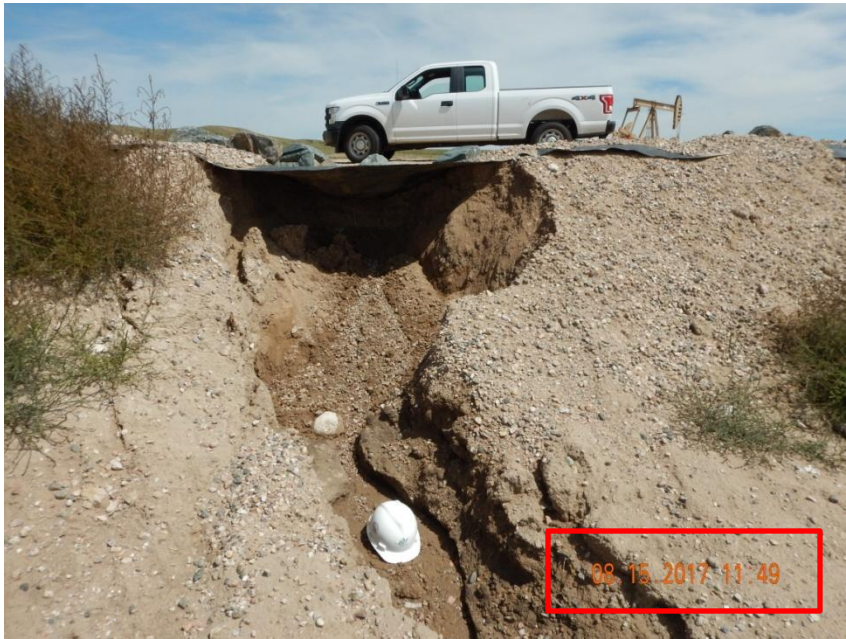
Photo 1. Photo taken on August 15, 2017 from the southwestern location, facing North. Gully erosion observed along the fill slope.
