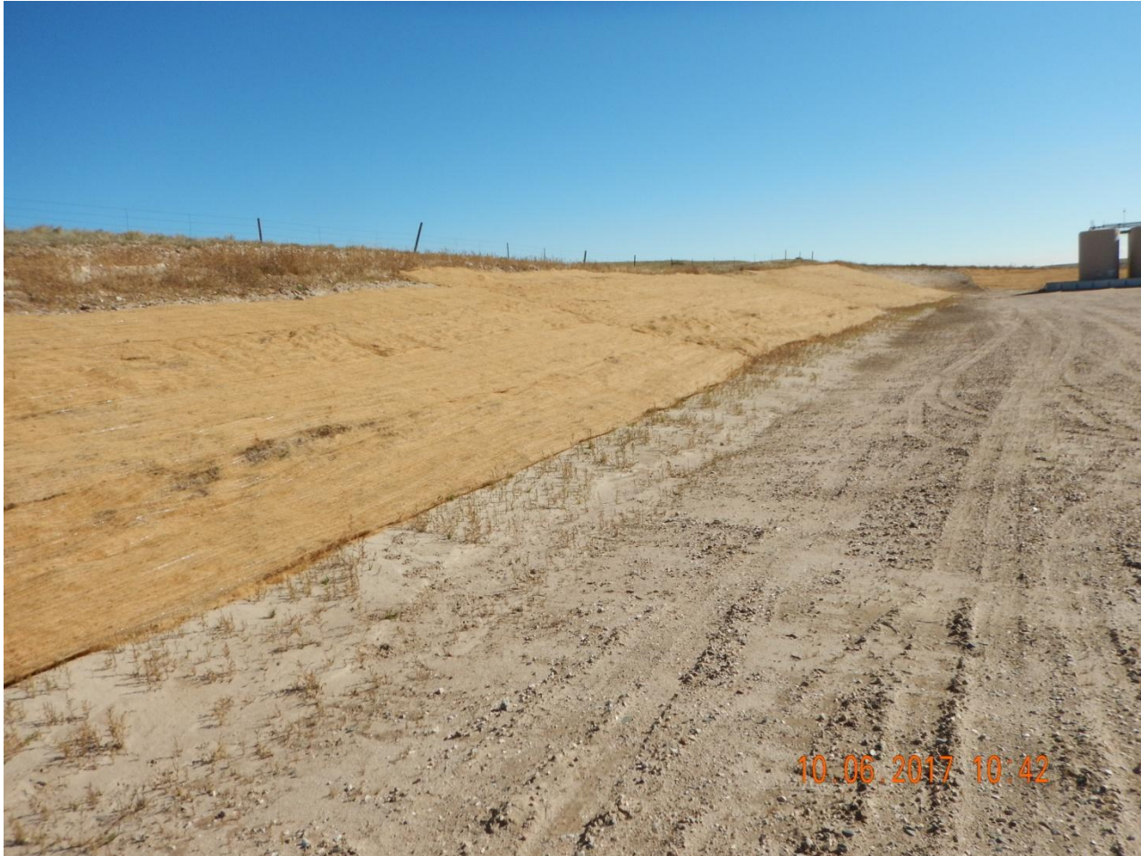
Photo 8. Photo taken from the northwestern cut slope area, facing East. Appears the Operator has installed erosion blankets along the entire cut slope; however, the Operator has not properly installed the BMP- see Photos 9-12.
