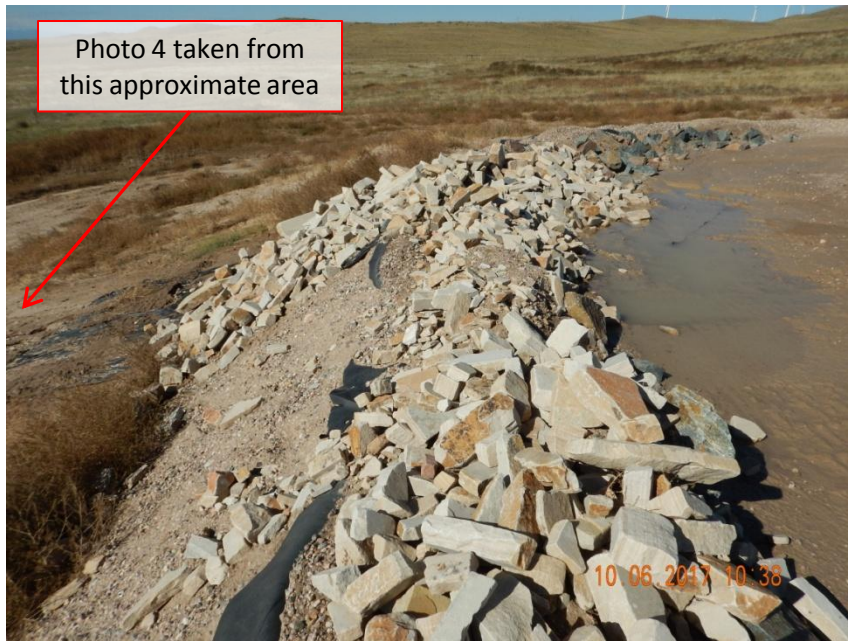
Photo 3. Photo taken from the southwestern location, facing West. Operator has haphazardly installed rock material that appears to be used as a berm BMP but appears to be functioning like a check dam- see Photo 4.
