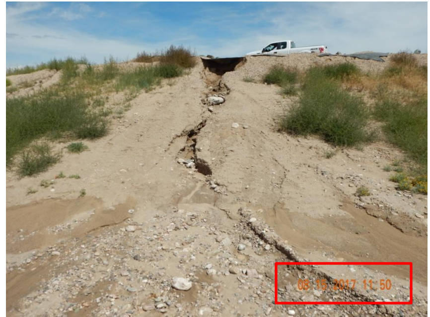
Photo 2. Photo taken on August 15, 2017 from the southwestern location, facing North. Gully erosion observed along the fill slope. Photo illustrates sediment deposition accumulation.
