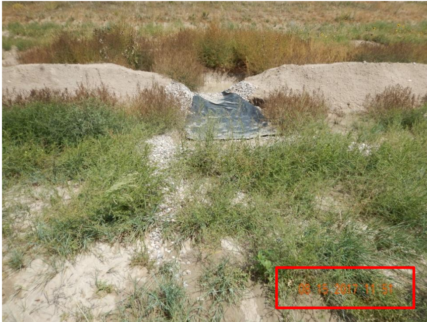
Photo 5. Photo taken on August 15, 2017 from the southwest sediment trap outlet area, facing North. Sediment trap does not appear to have a sufficient stabilized outlet. Rock material does not appear to be the appropriate size and the plastic-like material only appears to allow stormwater flows to accelerate out of the sediment trap. A point of sediment discharge was observed south of the outlet area.
