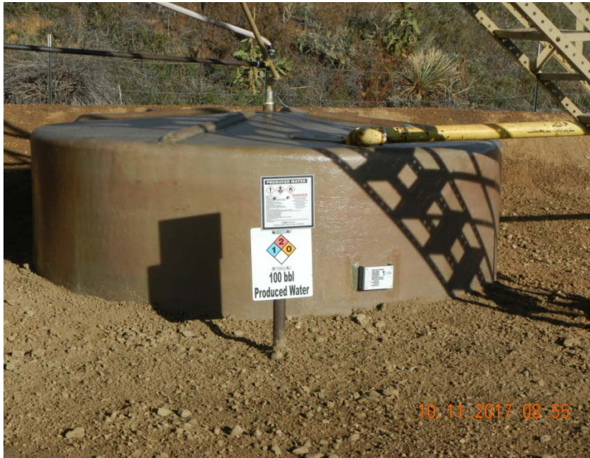
Replaced produced water vault
